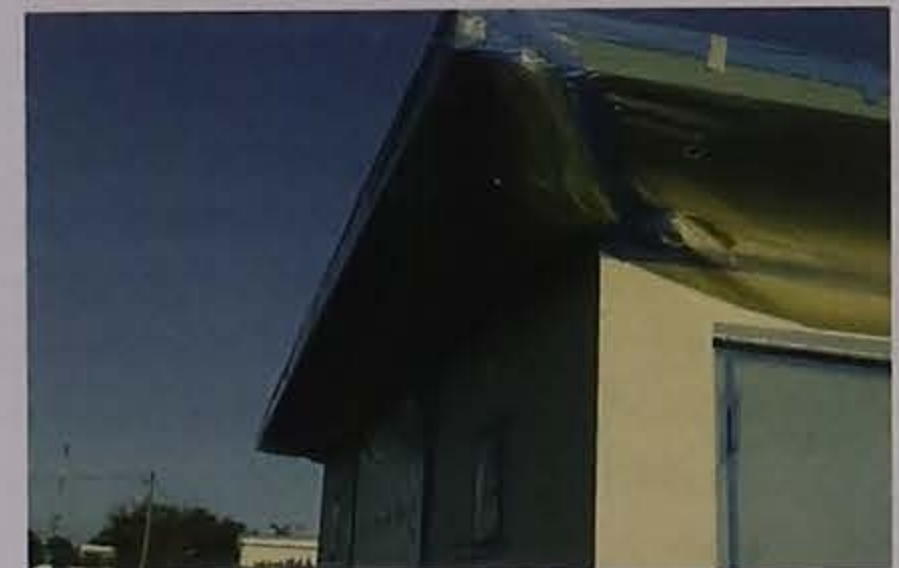
Figure 33. Tape-and-seal fumigation.
