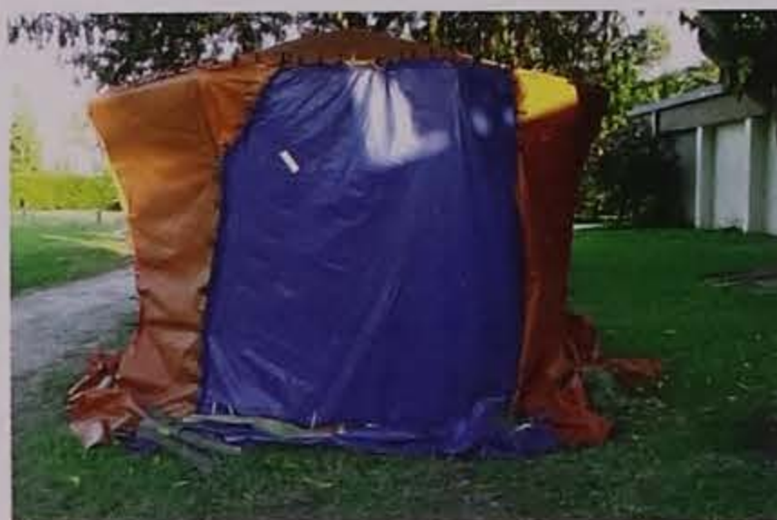
Figure 19. A sealed structure covered with vinyl-coated fabric tarps and weighted down with sand snakes.
