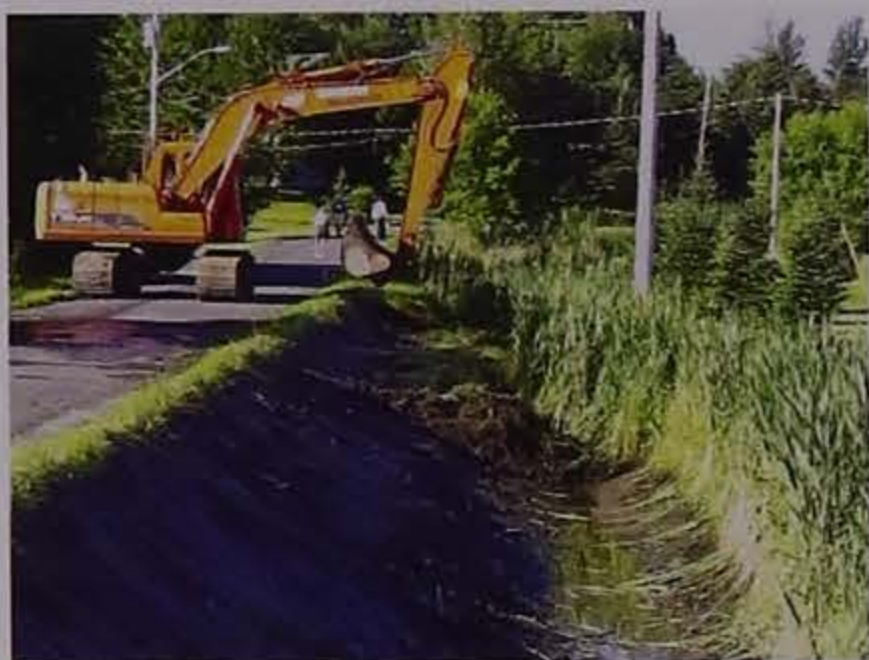
Figure 3.6. Cleaning roadside ditch to improve water drainage. Photo credit: Destinationknowlton.com
