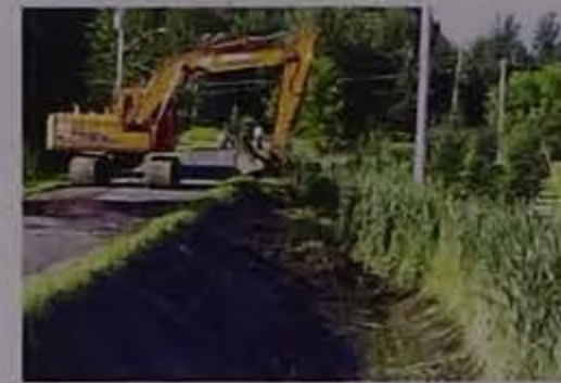
Cleaning a roadside ditch Destinationknowlton.com
