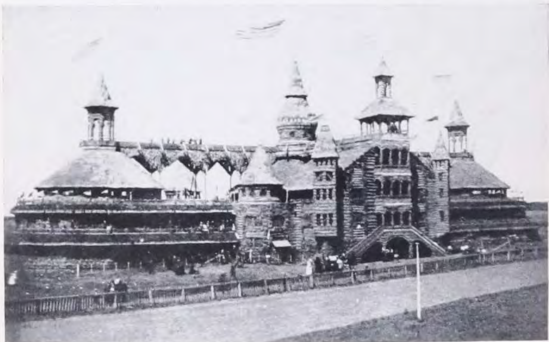
The "Bluegrass Palace," erected on the fair grounds near Creston in the fall of 1889 and enlarged in 1890, was 265 feet long and 130 feet wide. The main tower of the building was 120 feet high, with 90-foot towers on the wings and a 100-foot tower over the main entrance. Baled hay was used for gateways, for all projections and towers, and for the horseshoe arch at the main entrance. —CHAPTER 5, FORAGE CROPS THAT FEED THE LIVESTOCK AND SAVE THE SOIL.
