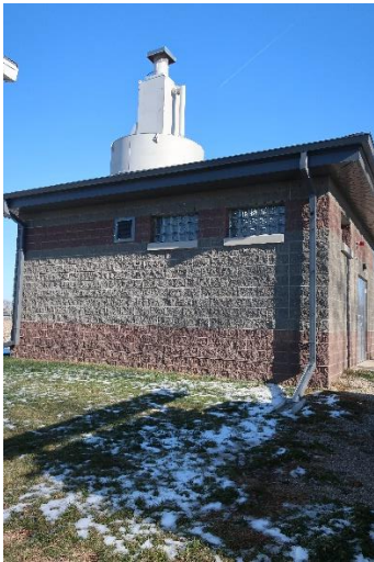
New water treatment plant building with aerator
