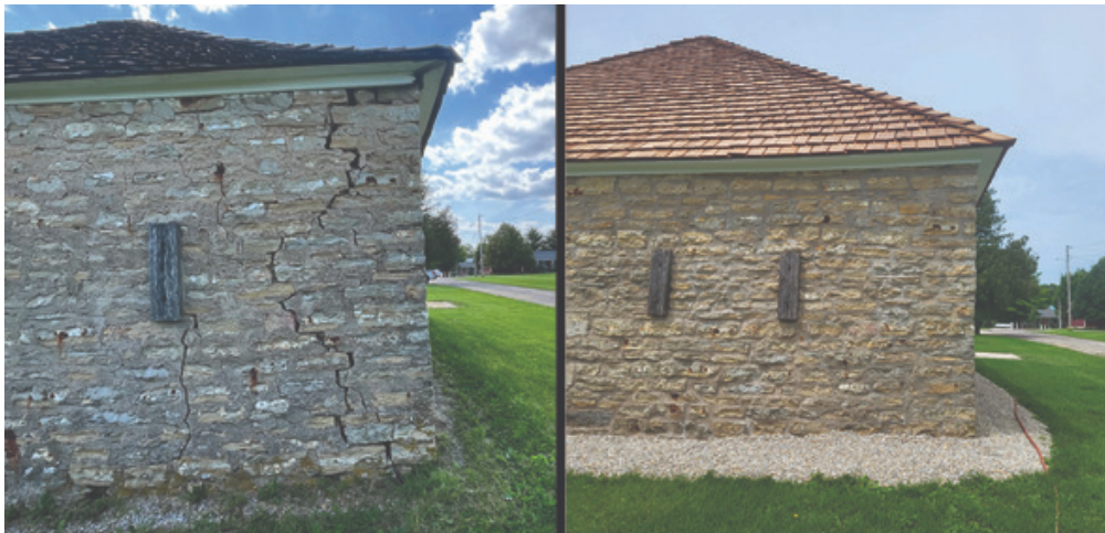
LEFT: Northeast Blockhouse at Fort Atkinson State Preserve with stone walls and roof in disrepair. RIGHT: Northeast Blockhouse with stone walls repaired and stabilized and roof replaced.
