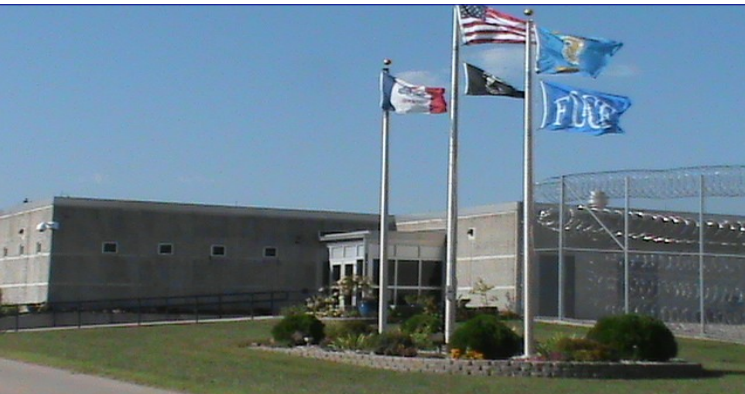
Fort Dodge Correctional Facility, Fort Dodge
