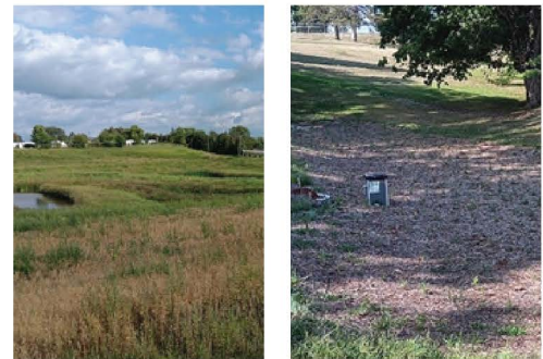
Stormwater wetland and bioretention cell in Waukon
