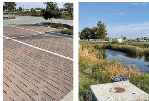
Permeable pavers and a bioretention cell in Waukee
