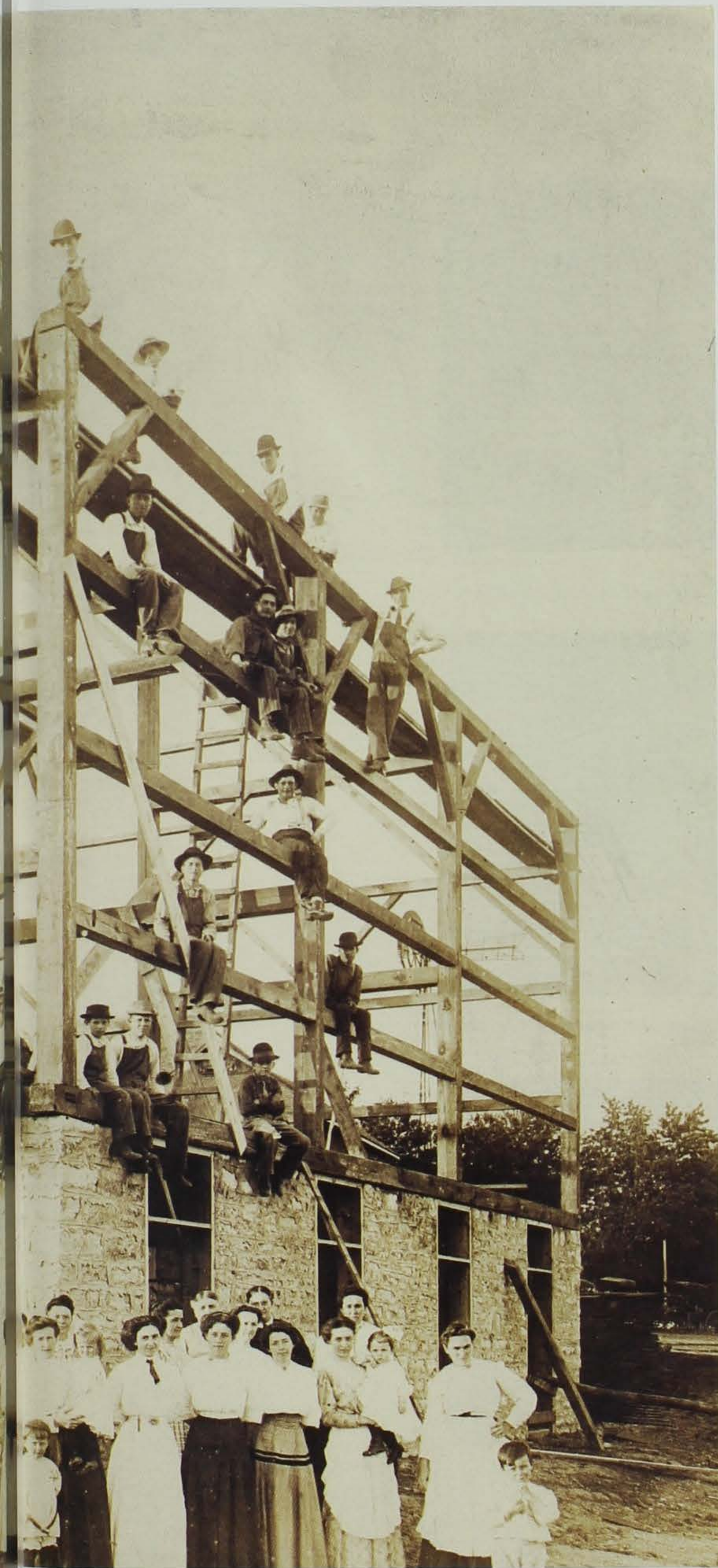
AN EARLY 20TH CENTURY BARN- RAISING NEAR HOLY CROSS, DUBUQUE COUNTY
