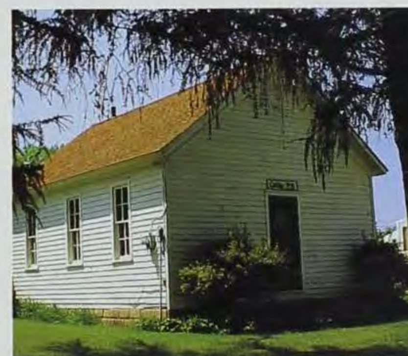
"UNCLE" HENRY WALLACE HOUSE, DES MOINES (TOP); AMERICAN GOTHIC HOUSE IN ELDON, WAPELLO COUNTY (MIDDLE); HERBERT QUICK SCHOOL- HOUSE IN GRUNDY CENTER, GRUNDY COUNTY (BOTTOM)
