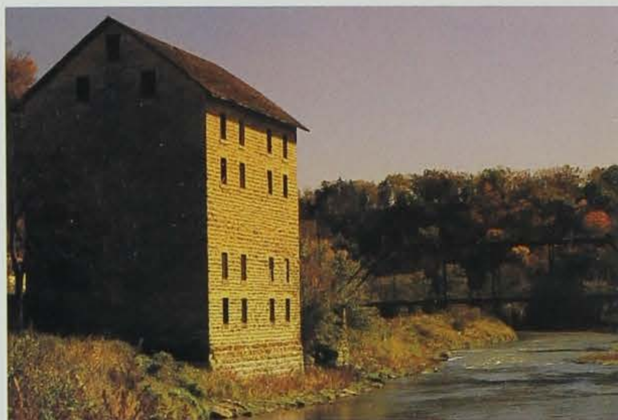
OLD MILL ON TURKEY RIVER, ELKADER, CLAYTON COUNTY
