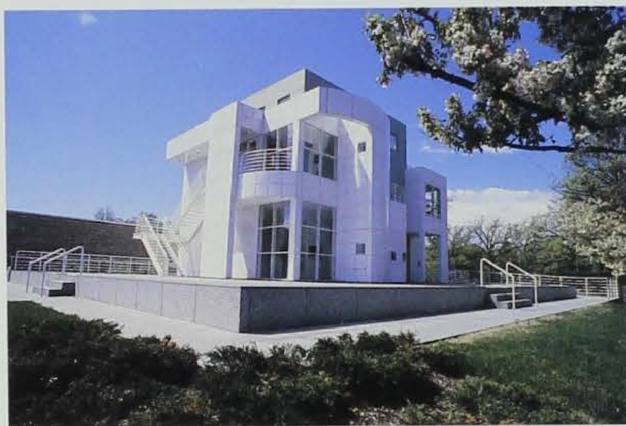
DES MOINES ART CENTER RICHARD MEIER ADDITION, POLK COUNTY
