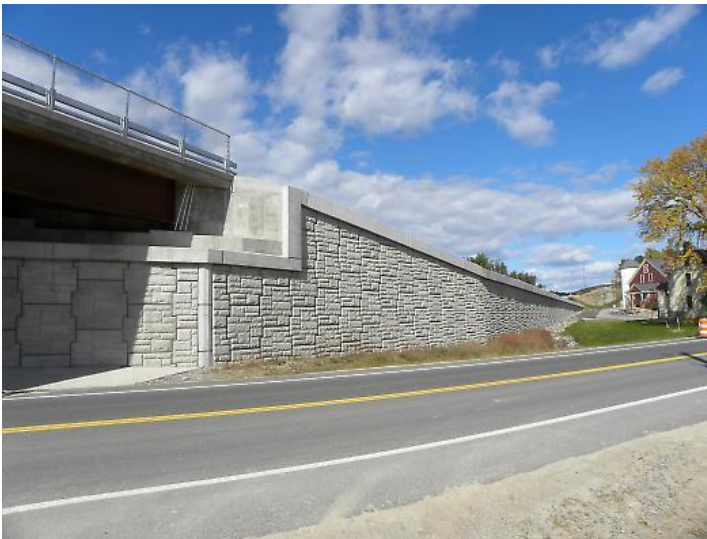
Figure 9 Example of a retaining wall
