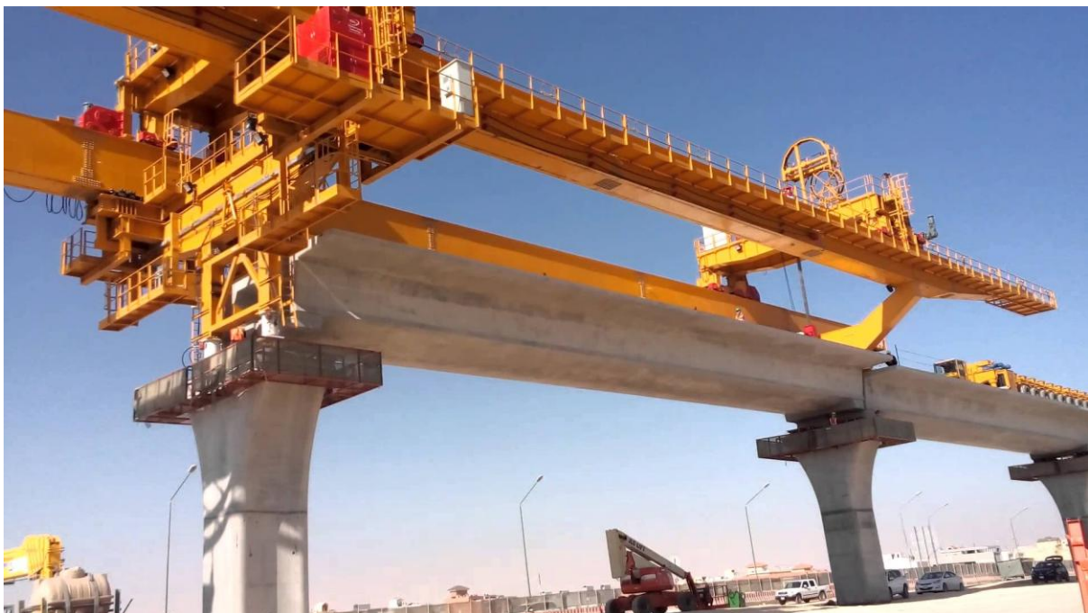
Figure 59 Example of a launching gantry
