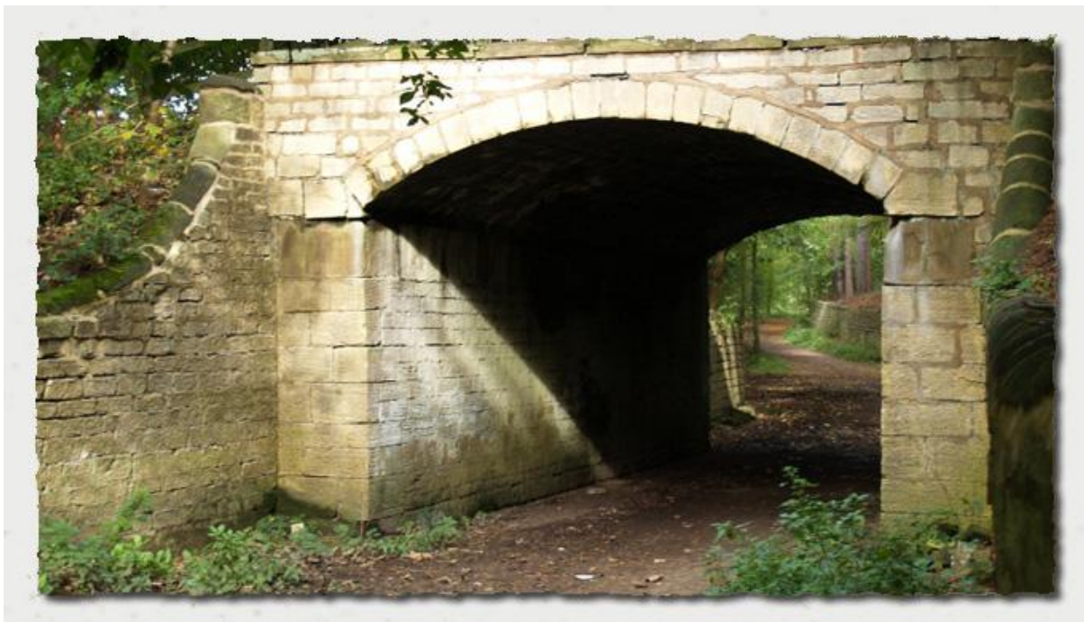
Figure 13 Example of a springer
