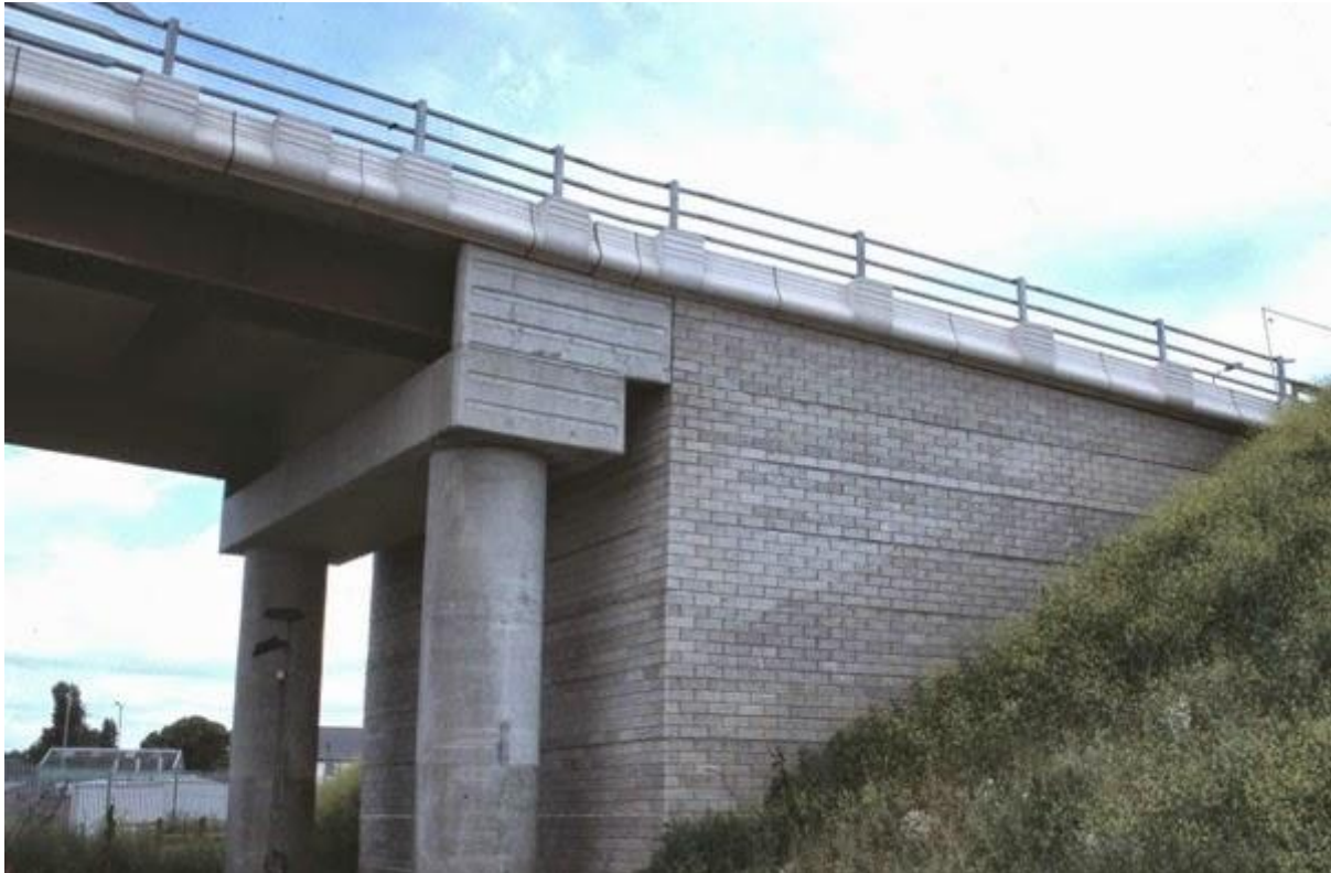
Figure 6 Example of an abutment
