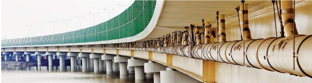
Figure 54 Example of a waste terminal
