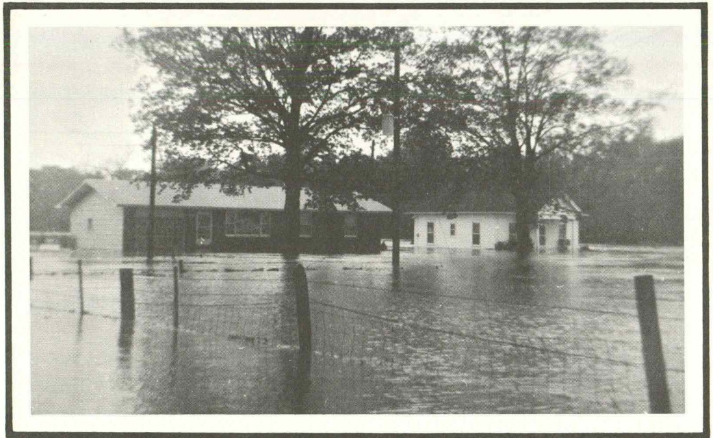
Figure 17. Looking southwest from Prairie Street during the flood of June 1967.
