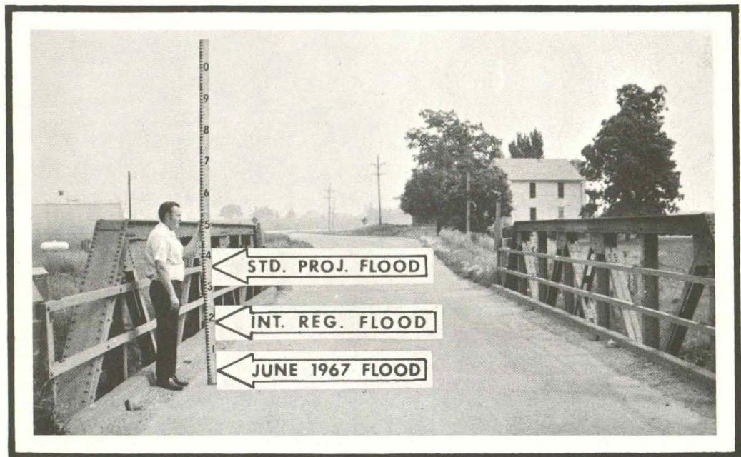
Figure 28. Upstream side of County Road X-40 bridge at mile 12.45 (Middle Branch), looking north.
