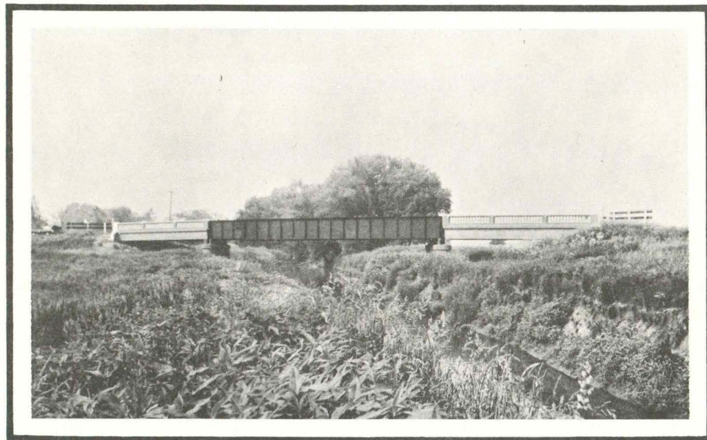
Figure 2. Iowa Highway 70 bridge at mile 9.35 (Wapsinonoc Creek), looking downstream.
