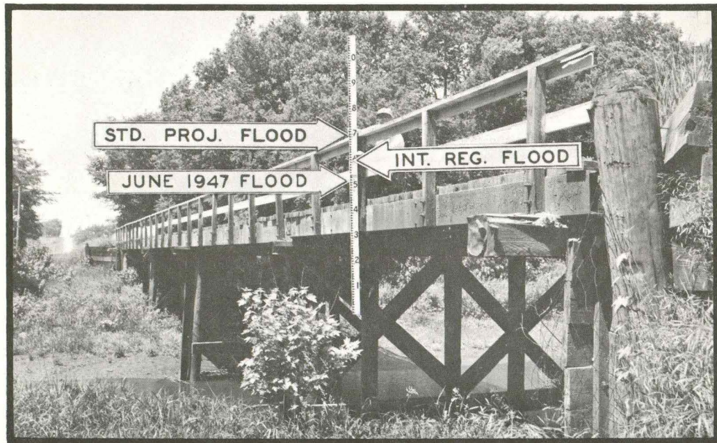
Figure 32. Downstream side of Ranchero Road bridge at Mile 5.30.
