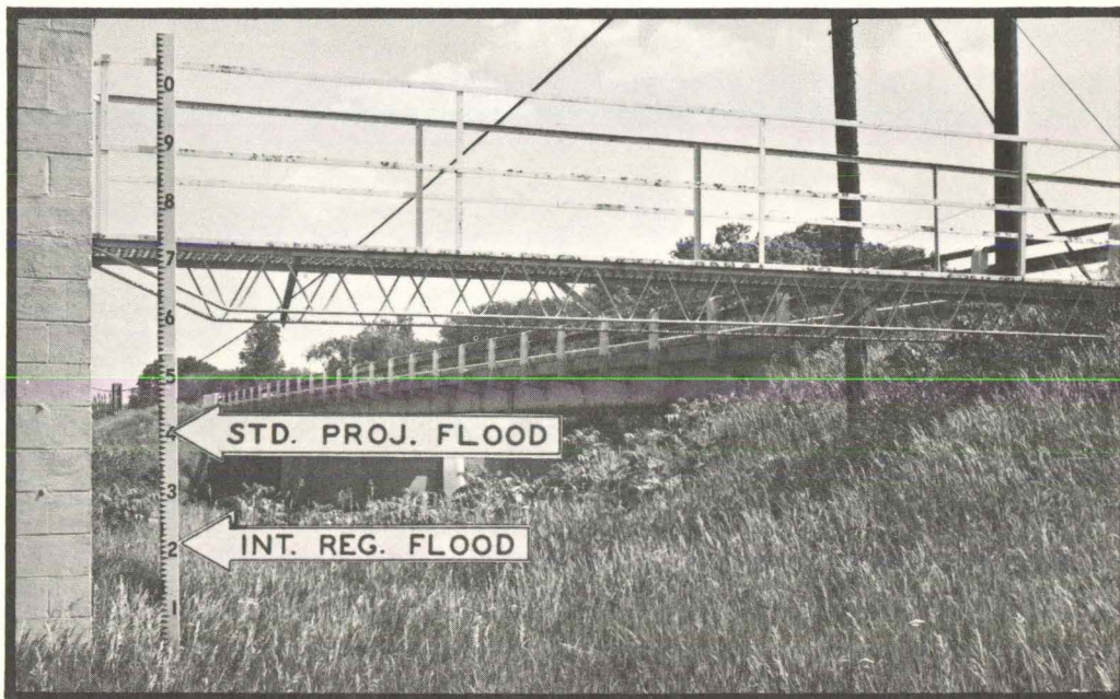
Figure 34. Downstream side of State Highway 58 bridge at Hudson Gaging Station - Mile 9.64.
