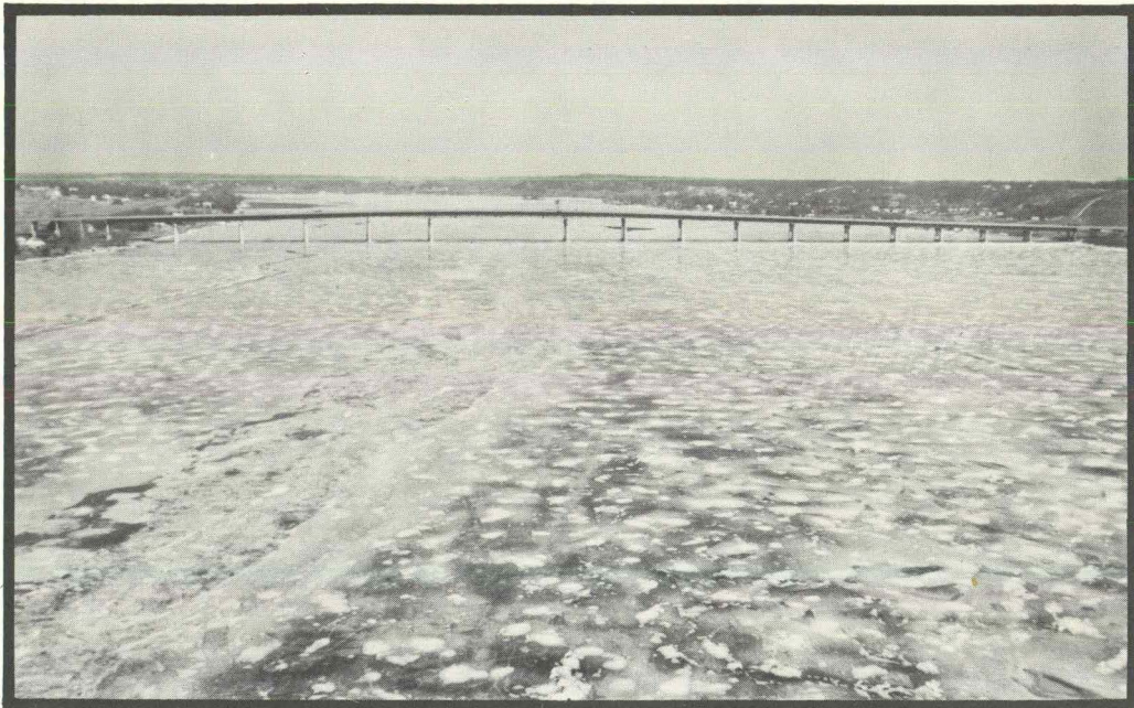
Figure 8. Looking upstream at the Interstate 80 dual bridges, Miles 495.4.
