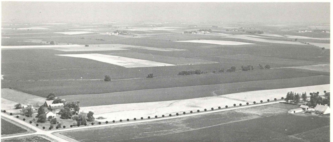
Low Angle Air View Shown from the Southeast Corner of the Site
