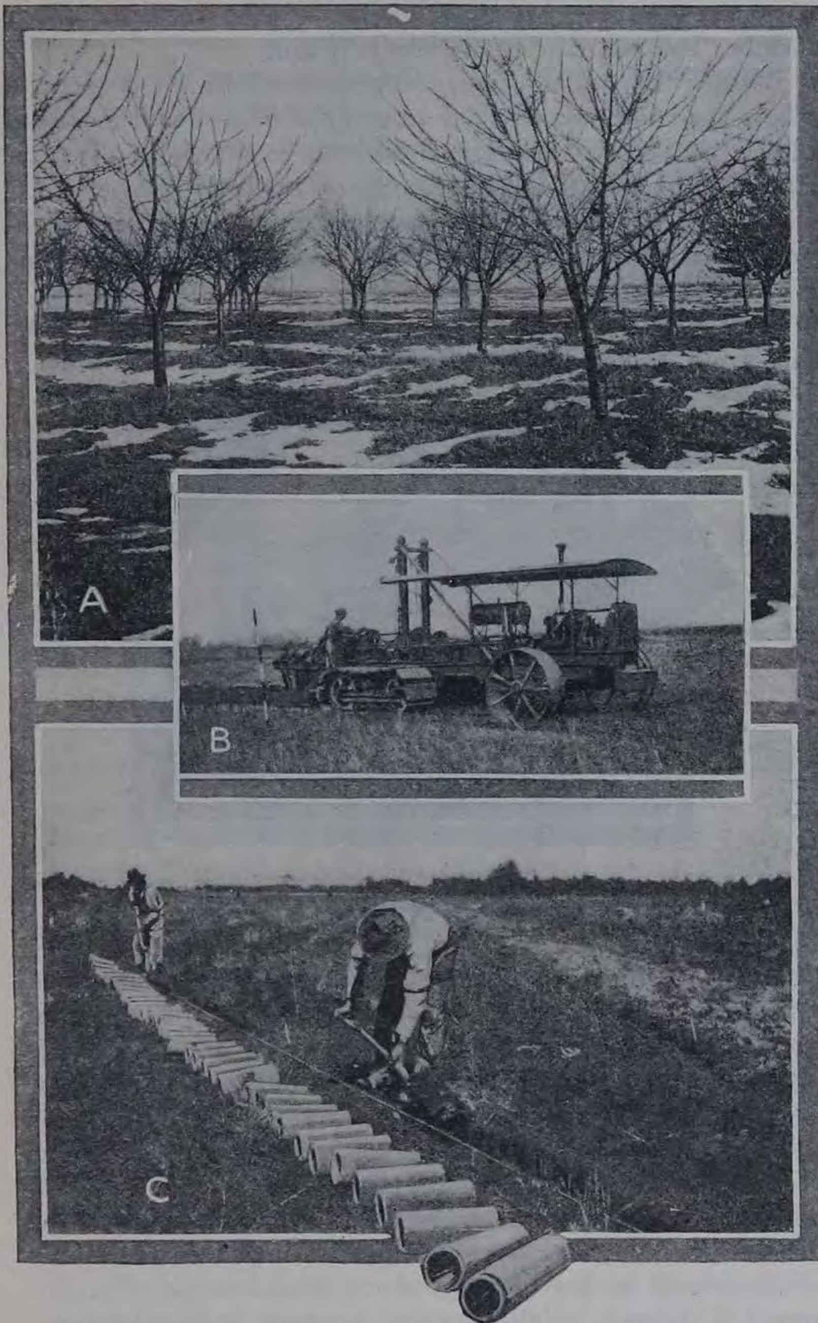
Two Methods of Ditching and Land Benefited by Drainage. A. Cherry orchard on Johnston farm. The land was tile-drained between 1835 and 1850. B. Community trenching machine at Hall, N. Y. C. Cutting trench with ditching spade.
