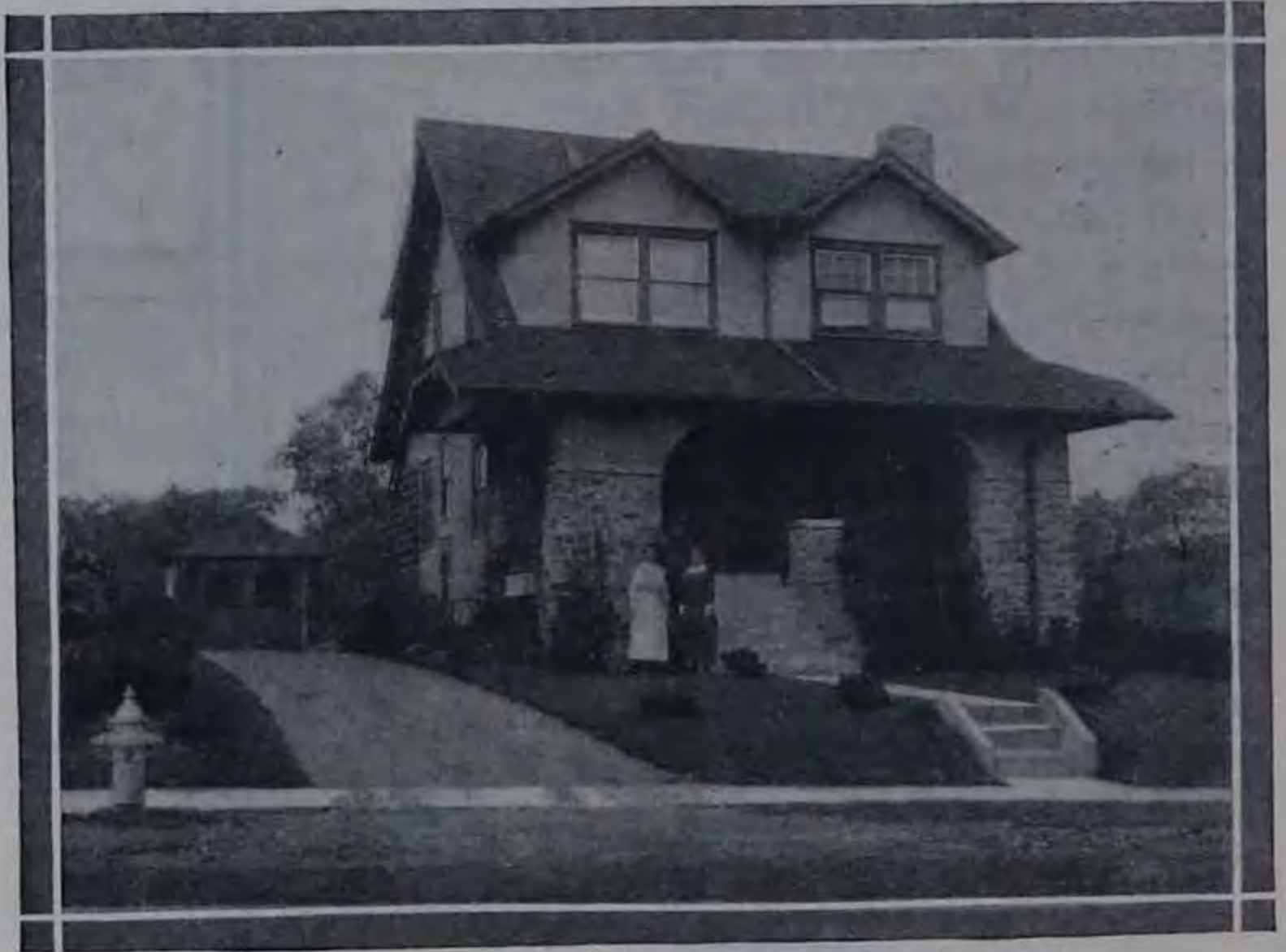
FIG. 8.—Where Roof Water Worked into the Cellar.
