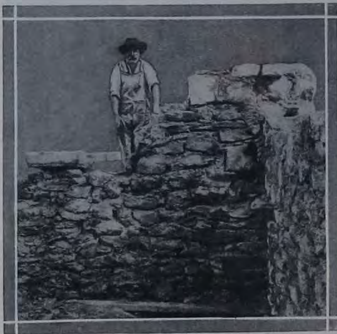
FIG. 3.—Inside Face of Wall Shown in Fig. 2.
