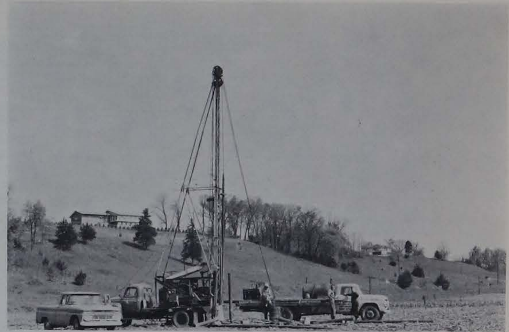
Water well being drilled into the alluvial aquifer of the Mississippi River Valley
