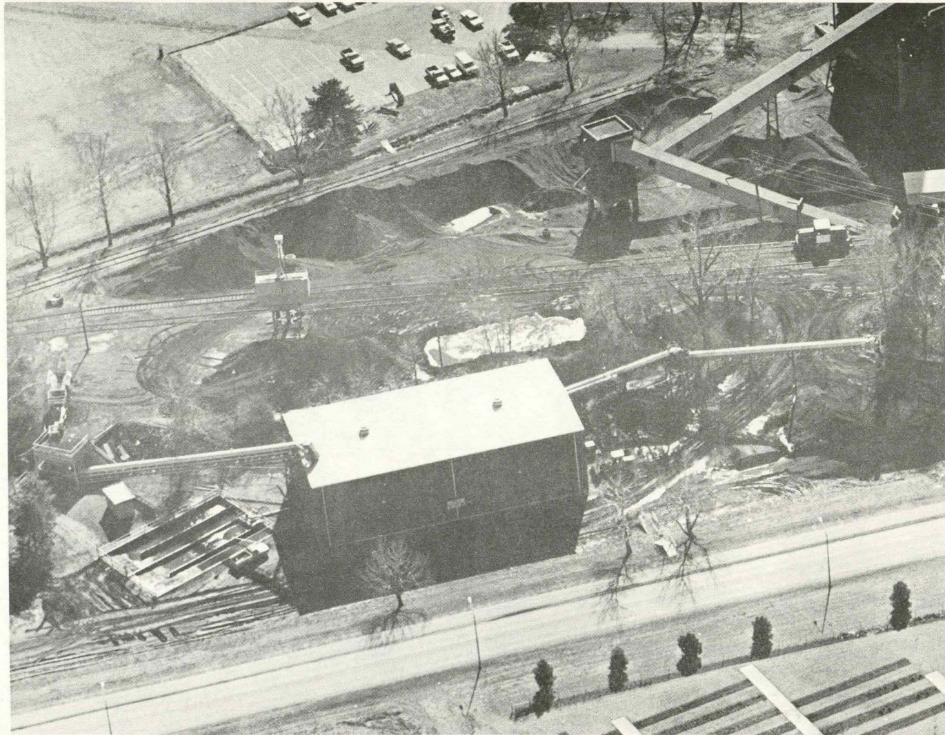
Figure 2. Aerial View of Iowa State University Coal Preparation Plant (white roof) showing close proximity to University Power Plant (Upper R.H. corner of photo)
