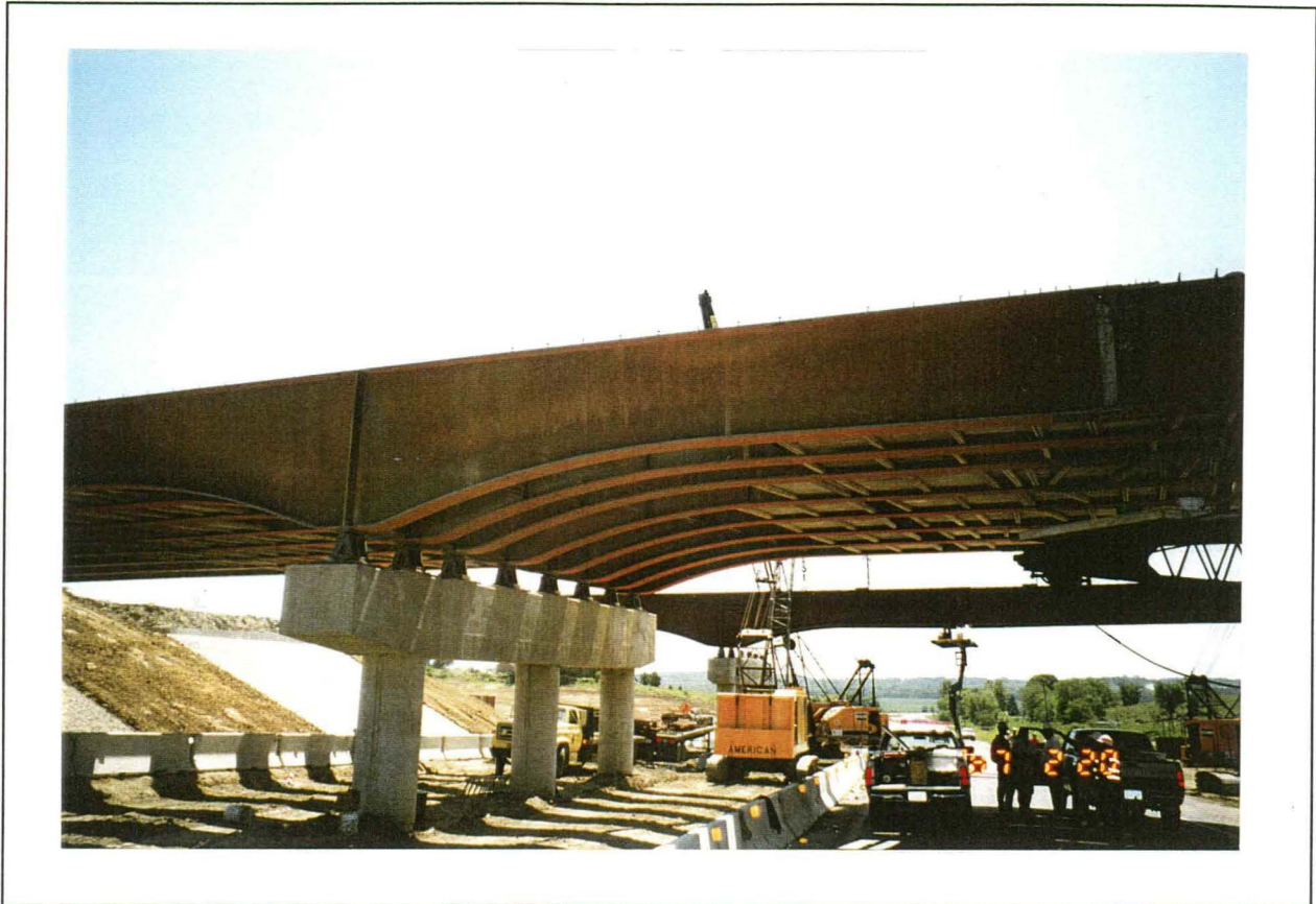
Figure 6 Haunched Steel Beams, Warren County, Iowa - IA 5 Bypass, Interchange with US 65 / 69
