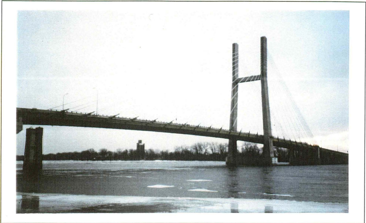
Figure 7 Cable-Stayed Bridge at Burlington, Iowa.
