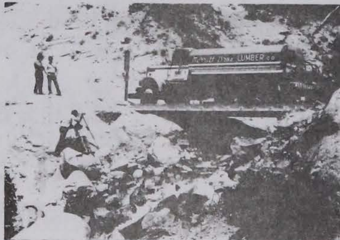
Figure 2. Load-testing an experimental stress-laminated bridge.
