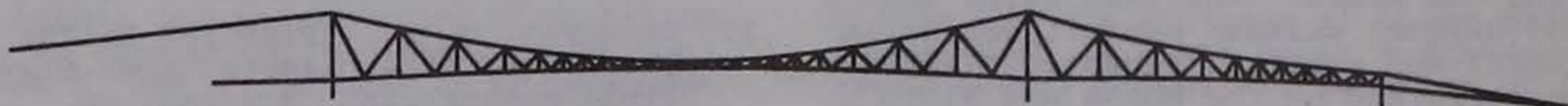
Figure 4 Missouri River Pipeline Suspension Bridge
