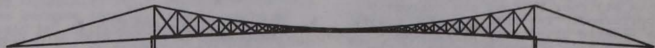
Figure 5 Mississippi River Pipeline Suspension Bridge
