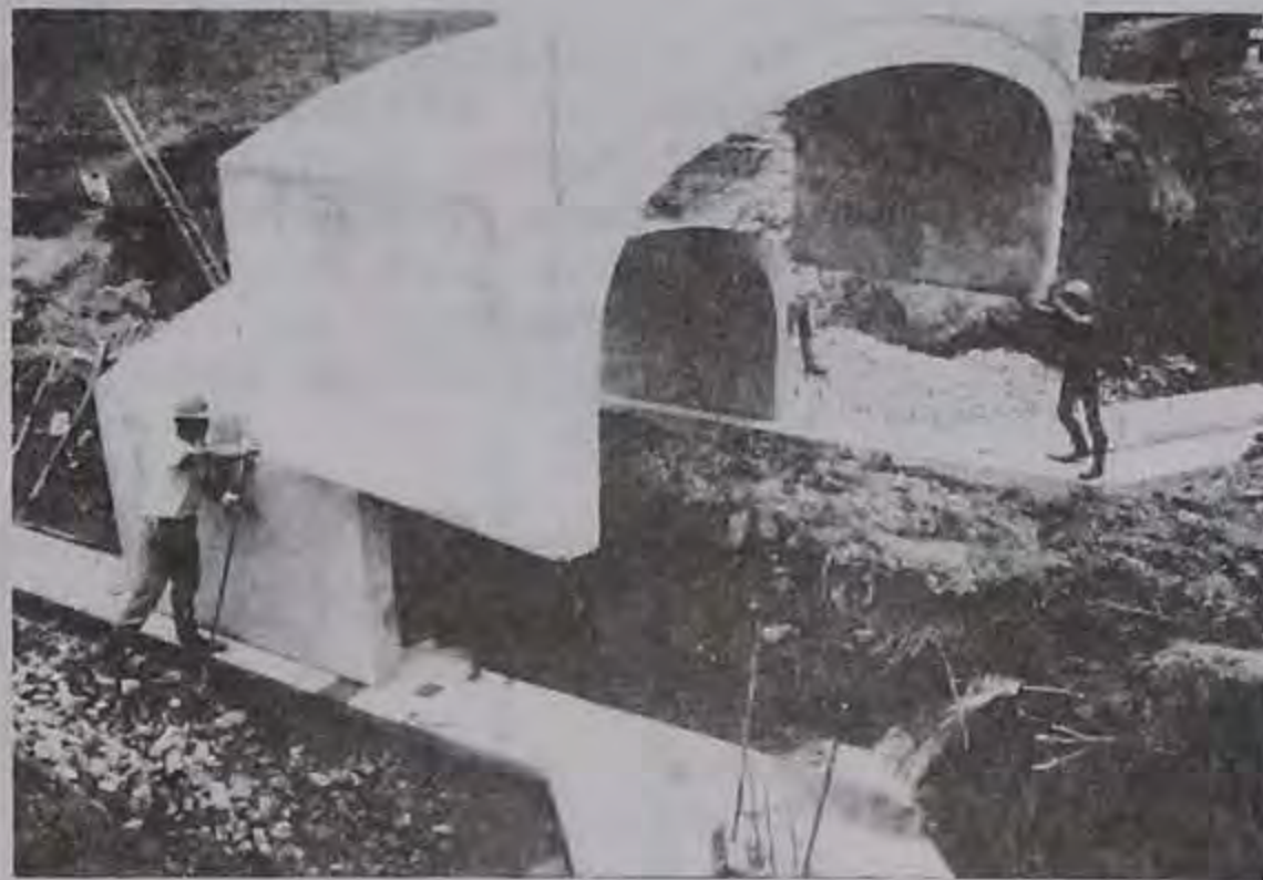
Figure 2. Setting pre-cast units.
