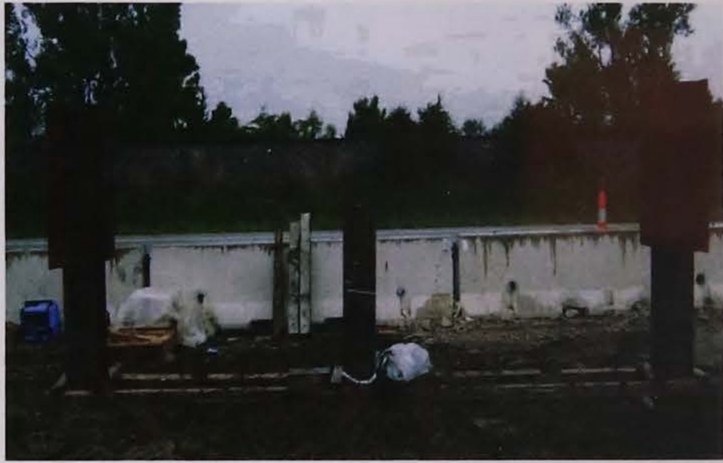
(b) A test pile between two anchored piles
