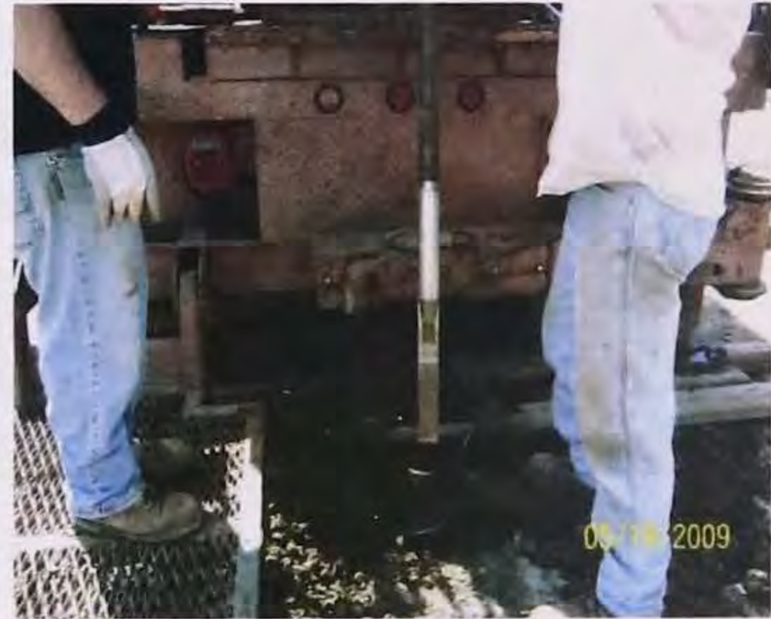
(b) Installing pressure cells
