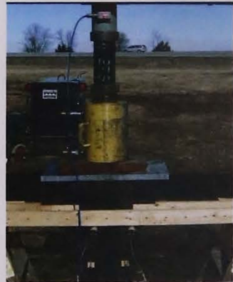
(d) Placed load cell and jack beams between test pile and beam
