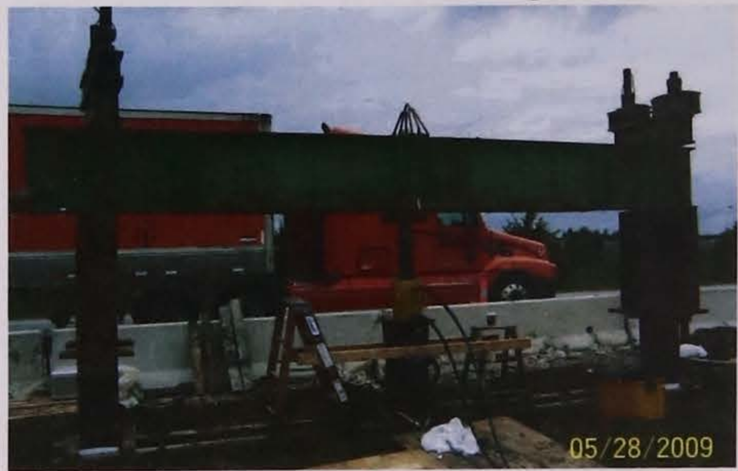
(f) Completed static load test frame
