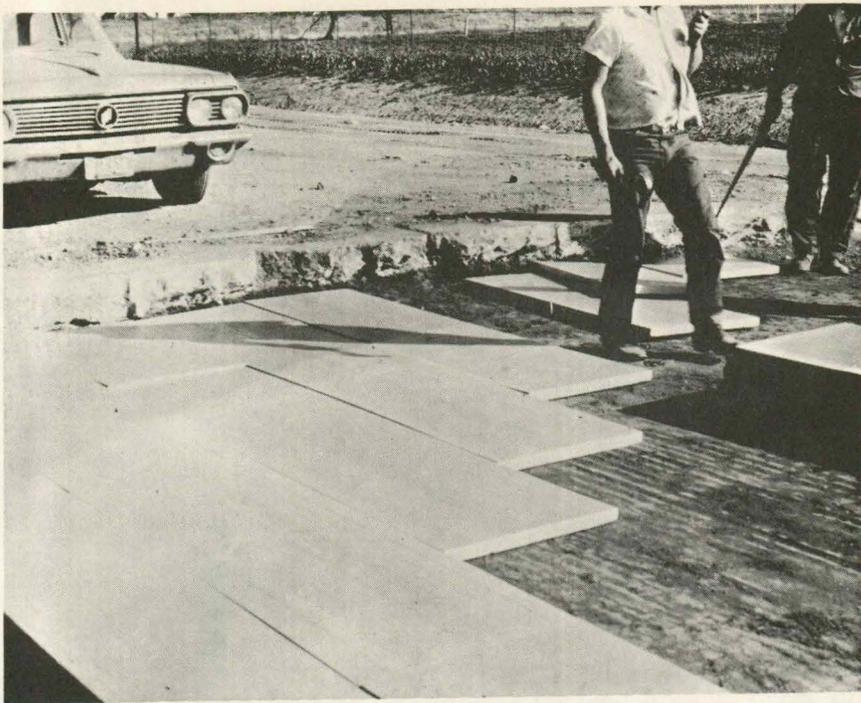
Photo 2: Placing 1½" Styrofoam on the Subgrade.
