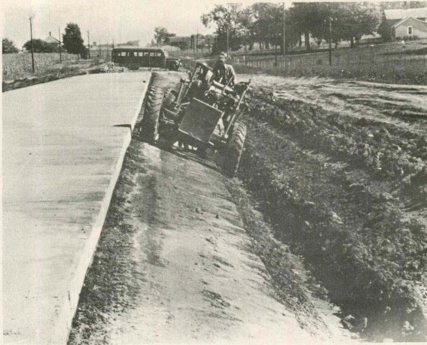
Photo 6: Cutting the 2:1 Shoulder Slope for the Styrofoam.
