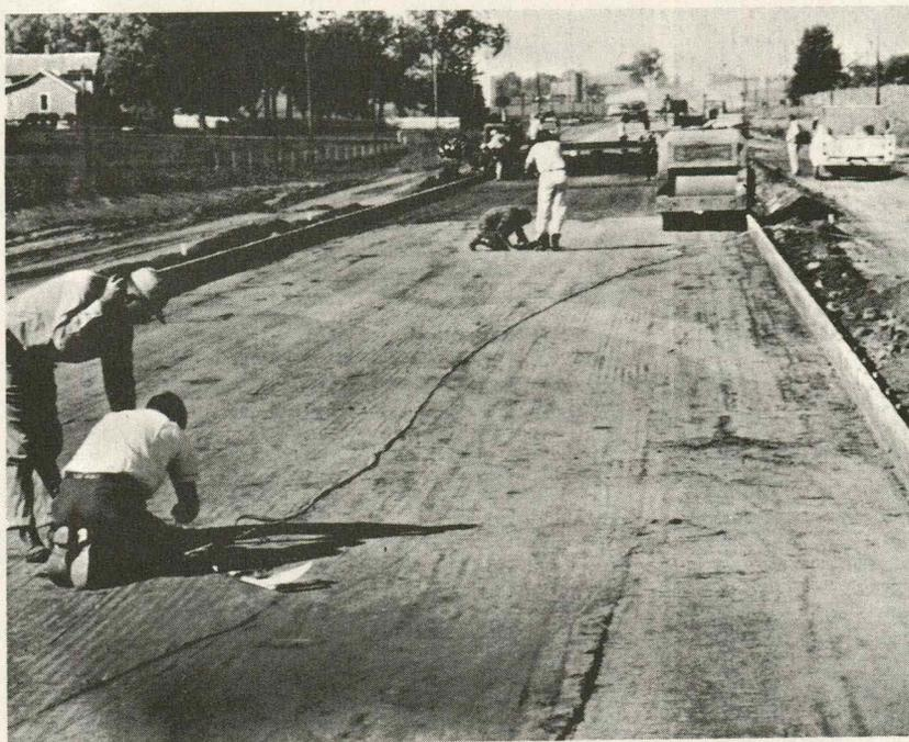
Photo 1: Installing the first thermocouple wires.
