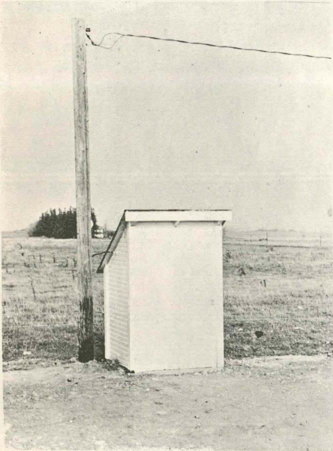
Photo 8: Housing for the temperature recording device.
