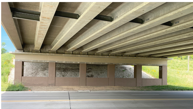
Instrumented frame pier of the 318 Scott bridge
