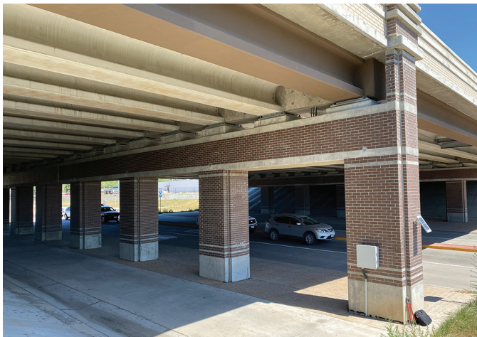
Instrumented frame pier of the 418 Woodbury bridge
