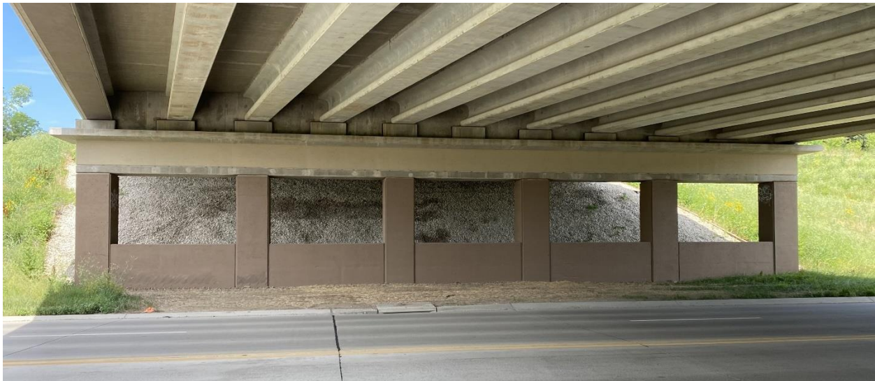
Figure 3.13. Instrumented frame pier of 318 Scott bridge
