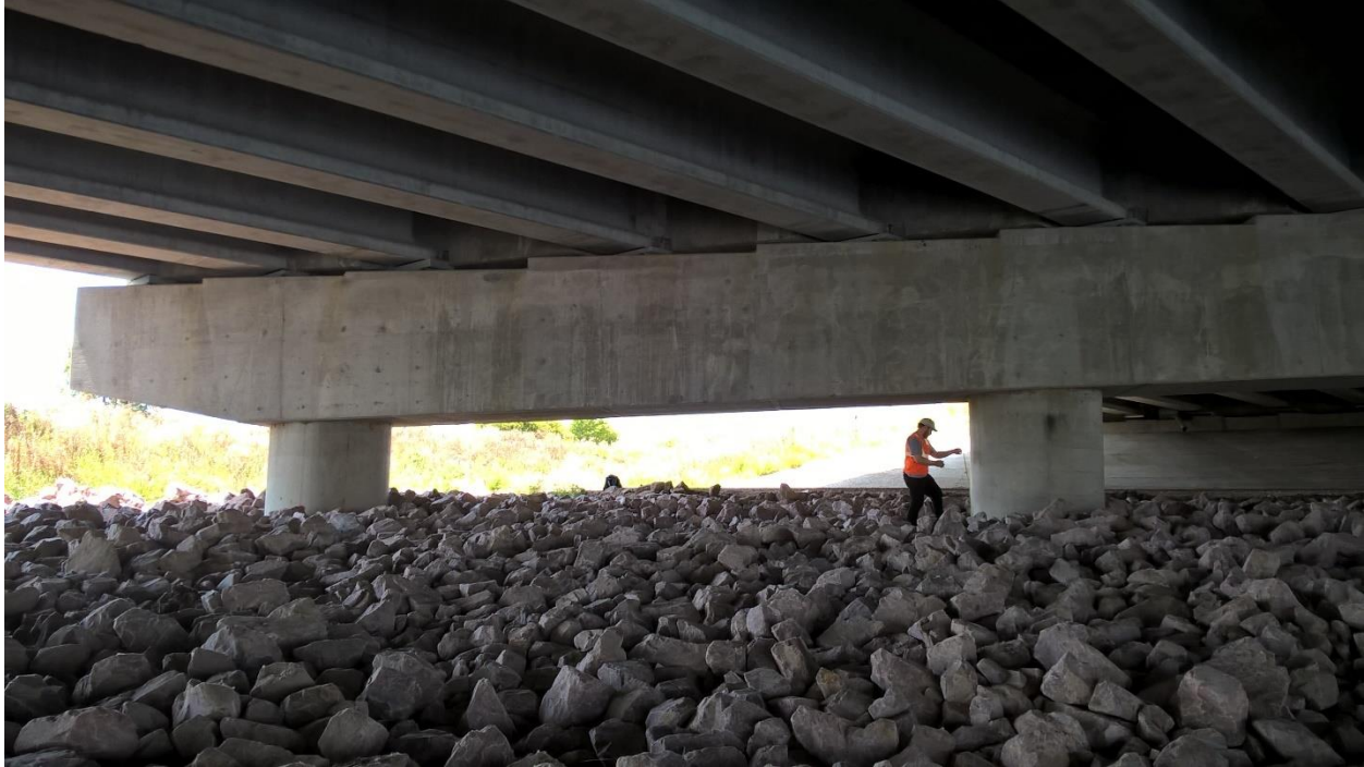
Figure 3.1. Inspected frame pier in Sioux City, Iowa
