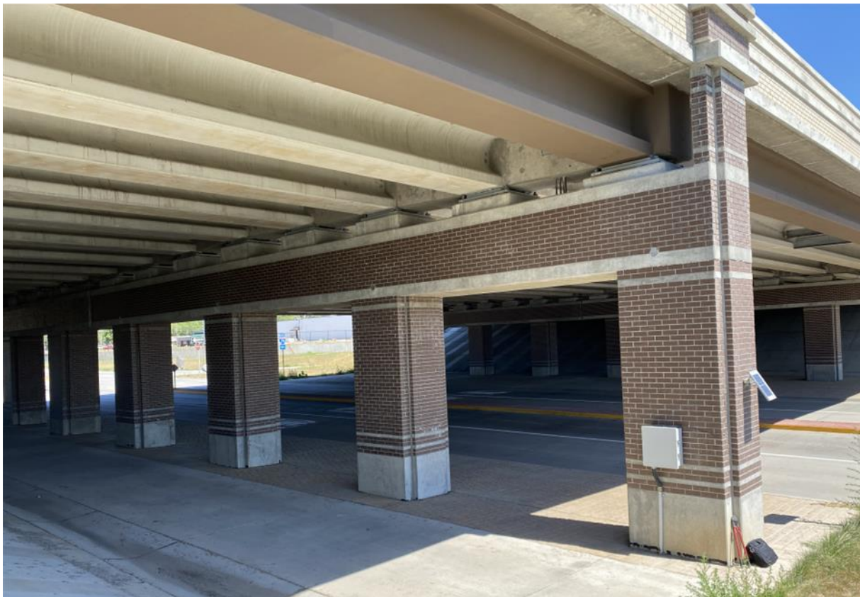
Figure 3.7. Instrumented frame pier of 418 Woodbury bridge
