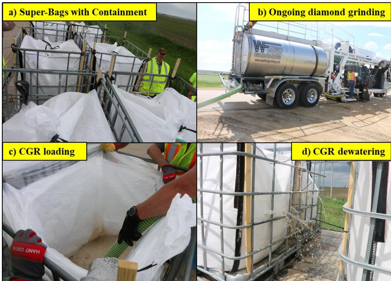
Figure 59. CGR collection at diamond grinding project site in Clinton County: (a) preparing the super bags with containment, (b) diamond grinding operations, (c) filling the super bags with CGR, and (d) dewatering the CGR bags
