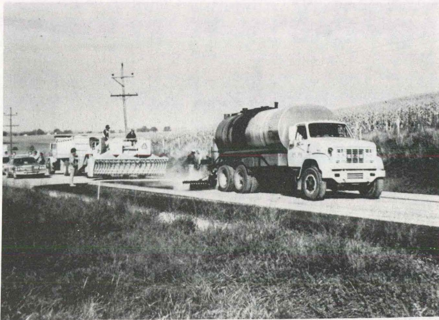
Tschiffgrie's equipment placing the seal coat.
