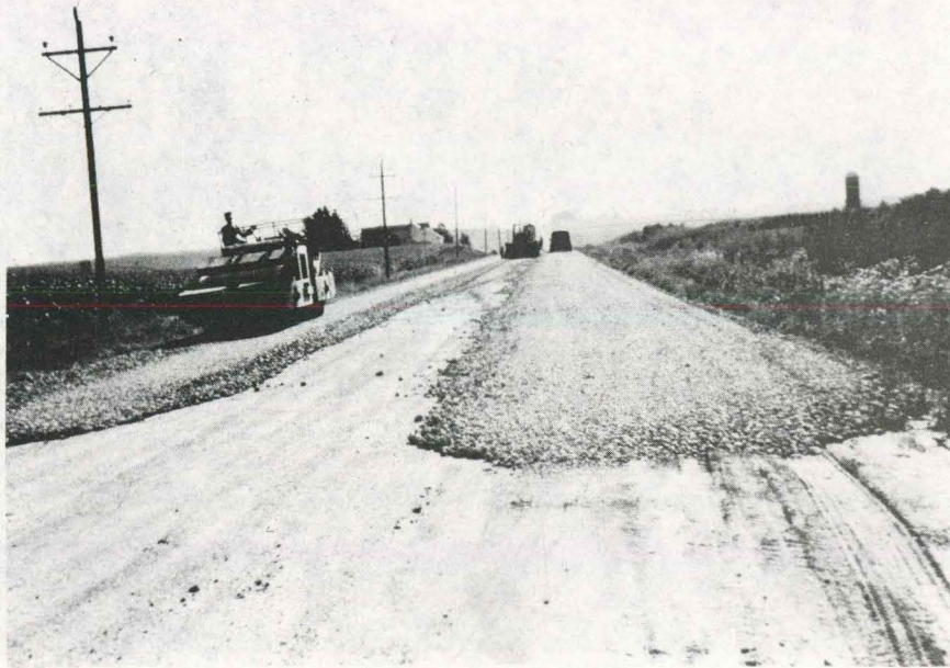
Plain macadam 6" base being placed.
