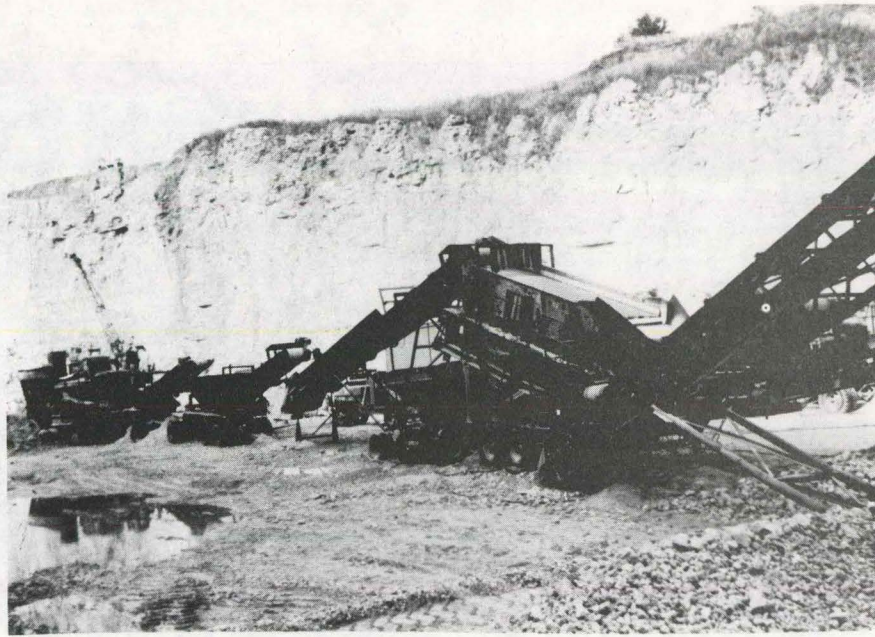
Meloy Quarry in Sections 22 and 23, T87N-R1E where Beecher LTD crushed the 3" macadam, 3/4" chokestone and the 3/4" class A stone.
