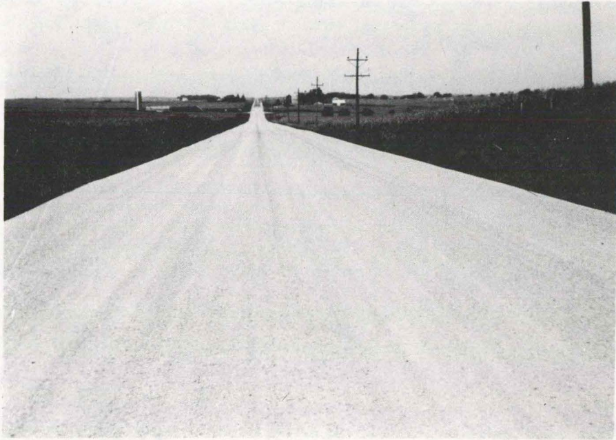
Section 6 with final seal coat looking easterly at station 131+00.
