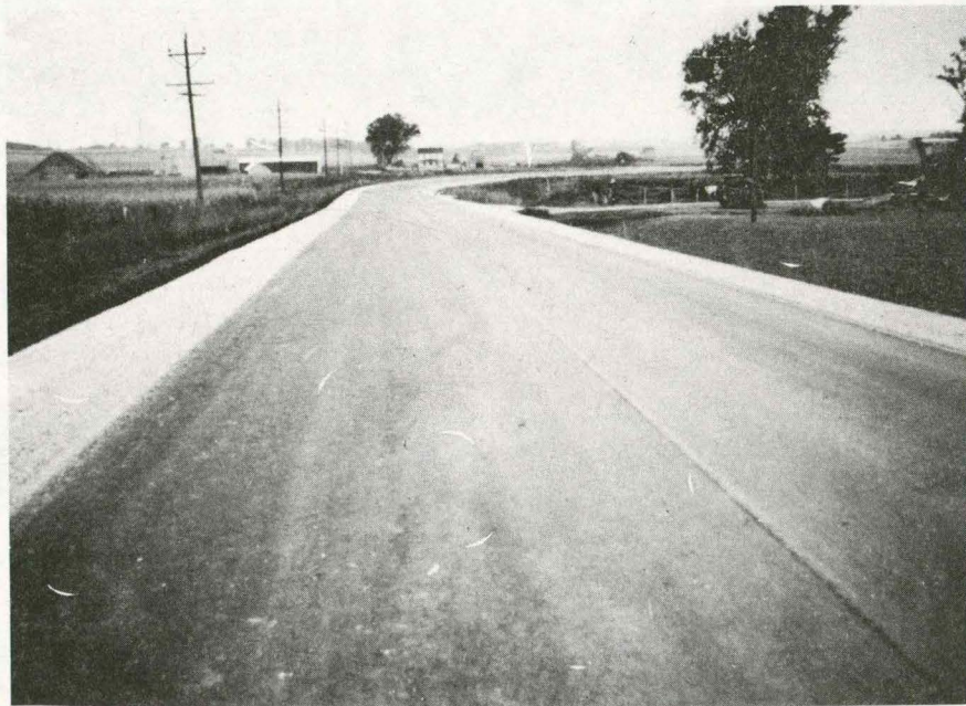
Final roadway. Section 3 looking westerly at Station 68+00.
