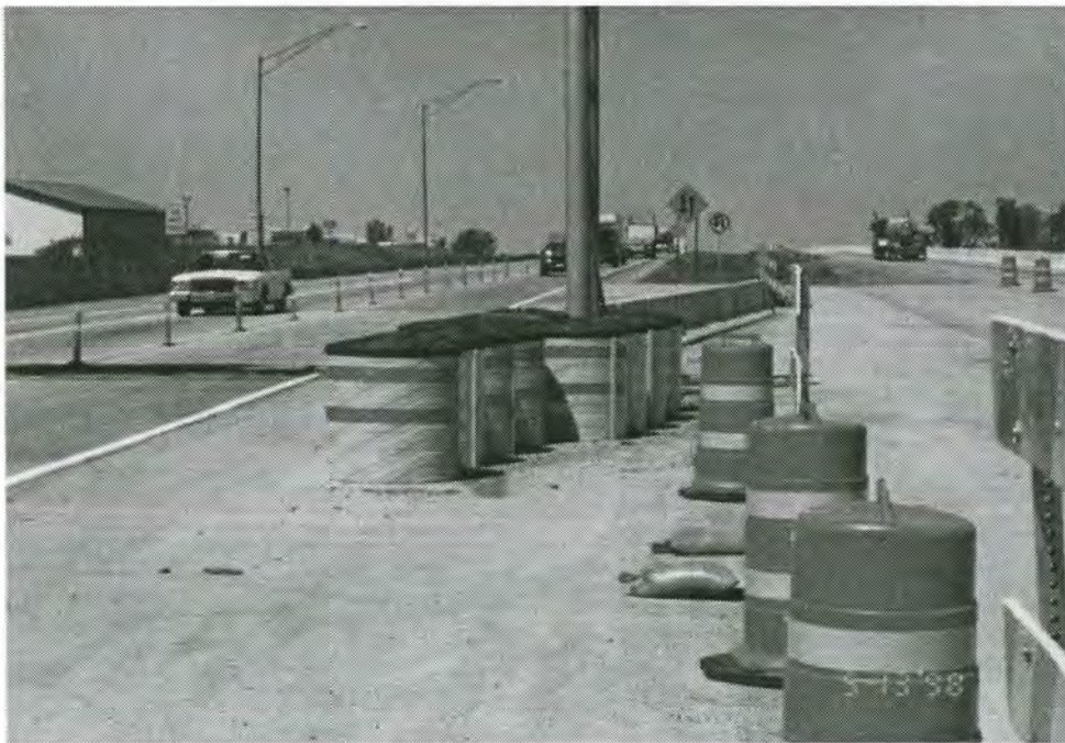
Figure 1: Sand-filled barrels may be used to shield obstacles in work zones.
