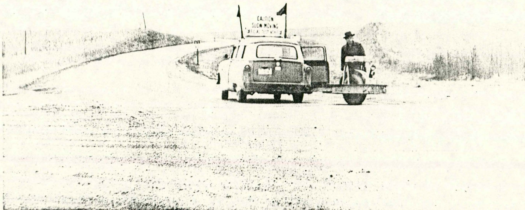
Figure 6. Resident Engineer at north end of slip-form project. Wheel of roughometer is located on Minnesota line.
