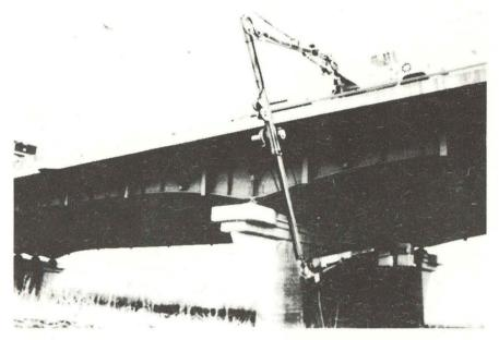
Each bridge is formally inspected biennially by bridge inspection crews and routinely by resident engineers for signs of deterioration in either the structure or deck. Routine repairs are performed by local bridge crews and repairs requiring specialized equipment are completed under contract.
