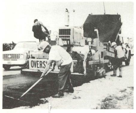
Each year approximately 85,000 manhours are used to place an average of 7,000 tons of premix to repair holes in the pavement surface. Machine leveling of the roadway to correct deterioration or uneven surface conditions require another 20,000 tons of material each year. Approximately 60 lane miles of roadway is burner-planed each year to correct heaved or wheel-rutted surfaces. This process will also increase surface traction by eliminating excess surface oils.
