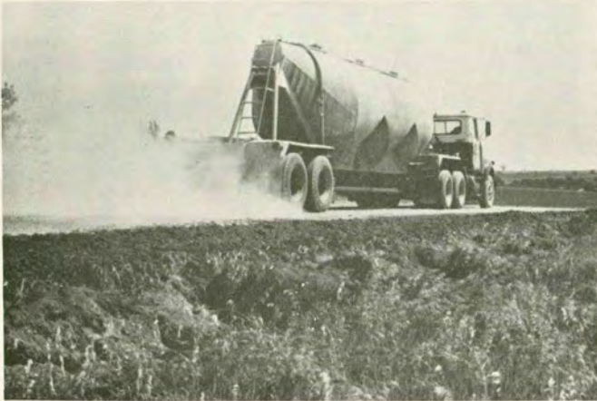
a. Cement spread.
