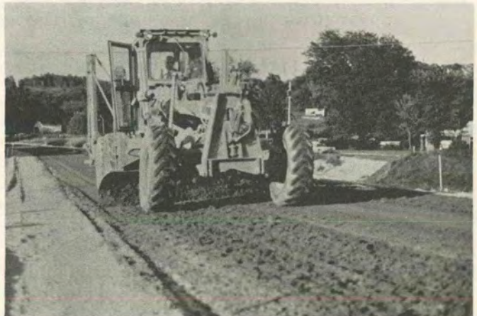
d. Final blading to known and cross-section following sheepfoot compaction.
