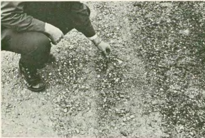
a. Section 1, CSSI asphalt emulsion.
