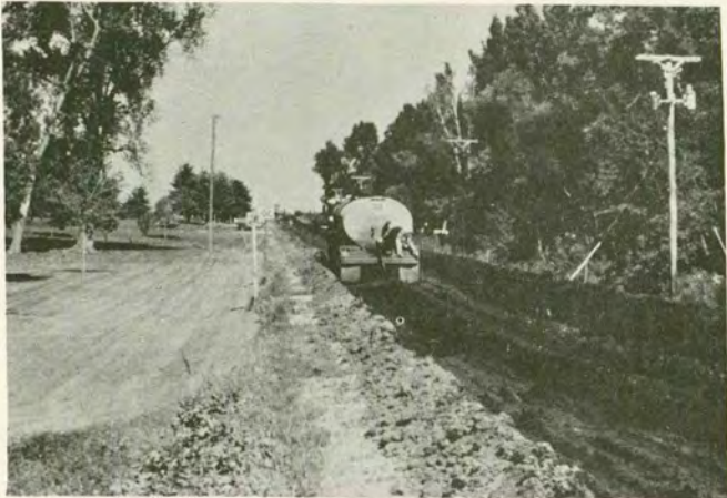
a. Asphalt emulsion application, section HC-2.
