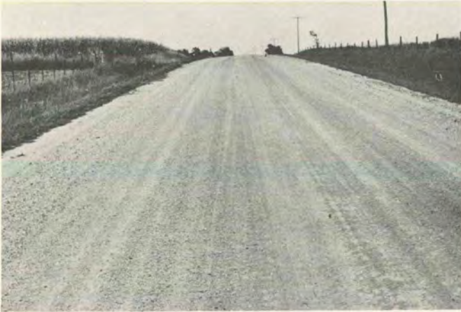
e. Section 6, Polybind Acrylic DLR 81-03.
