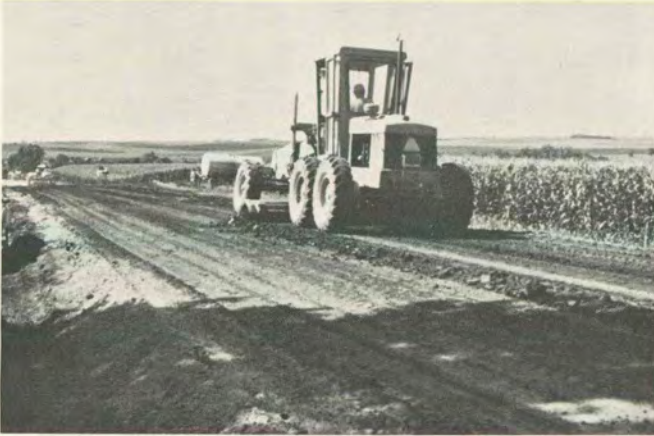
e. Final blading to crown, cross-section, and profile.
