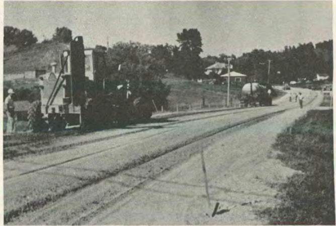
b. Addition of water (right), longitudinal mixing with blade (left).
