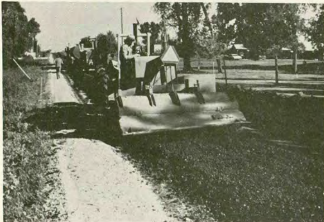
c. Rotary mixing, section HC-2.
