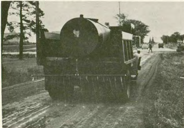
g. Second stage application of Coherex, October 16, 1980.
