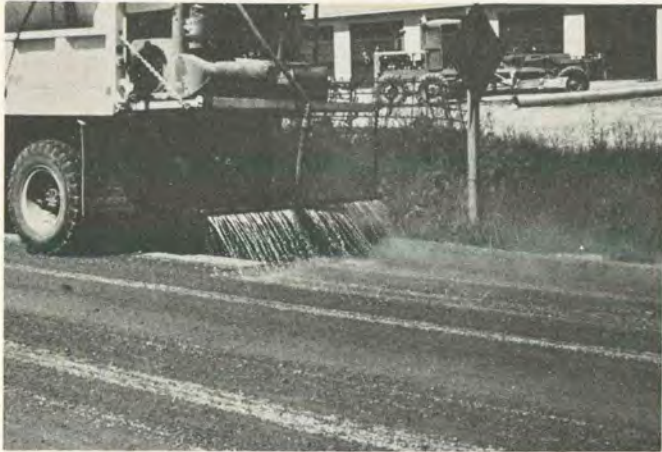
a. First surface spray application, section 2, August 21, 1980.
