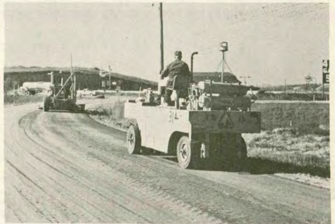
h. Finish blading and rubber tired compaction, section N-2.
