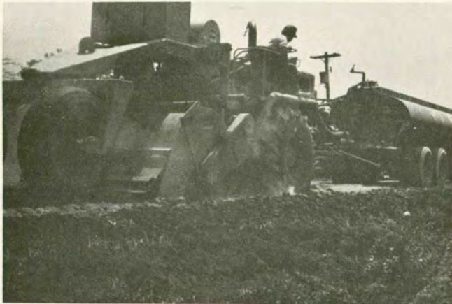
c. Final mixing, with water tanker direct feed to rotary mixer.
