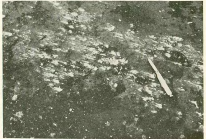
f. Surface condition following tight blading, October 16, 1980.
