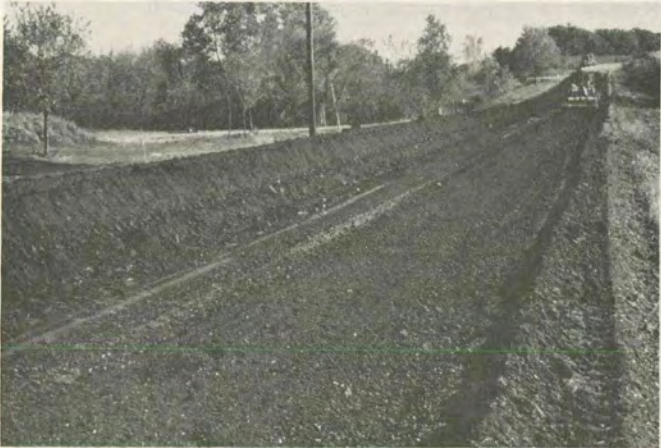
c. Mixed material windrowed (left), final mixing (right), section N-1.
