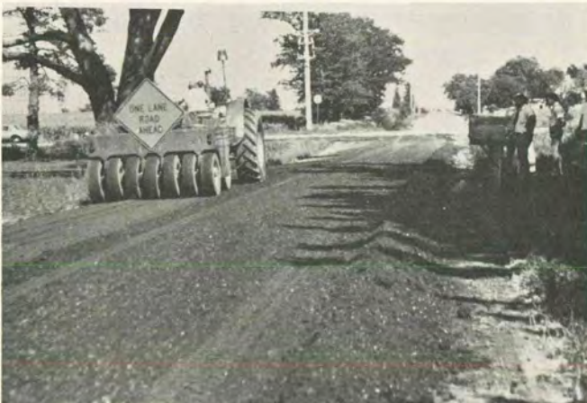
c. Rubber tired compaction.
