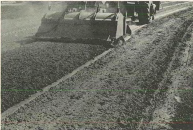
c. In-place mixing of cement and fly ash.
