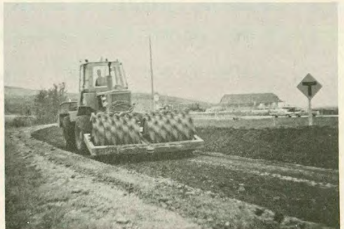
g. Tamping foot compaction, section N-2.
