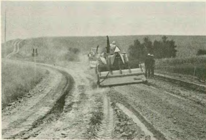
f. Rotary mixing, section N-2.
