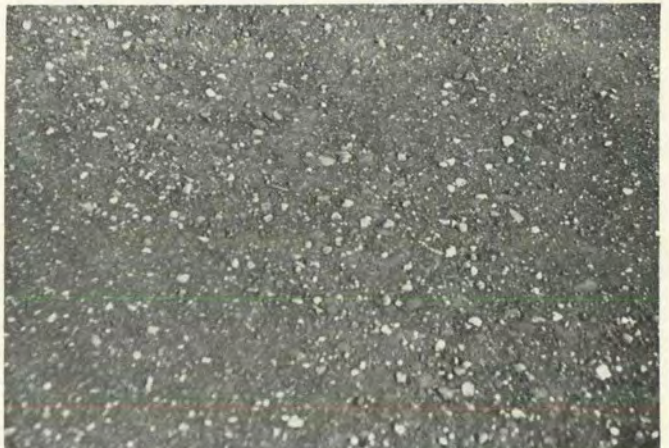
d. Surface condition, completion of construction, August 18, 1980.
