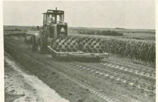
d. Tamping foot compaction.
