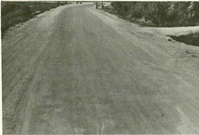
g. Finished roadway, new surface, August 26, 1980.
