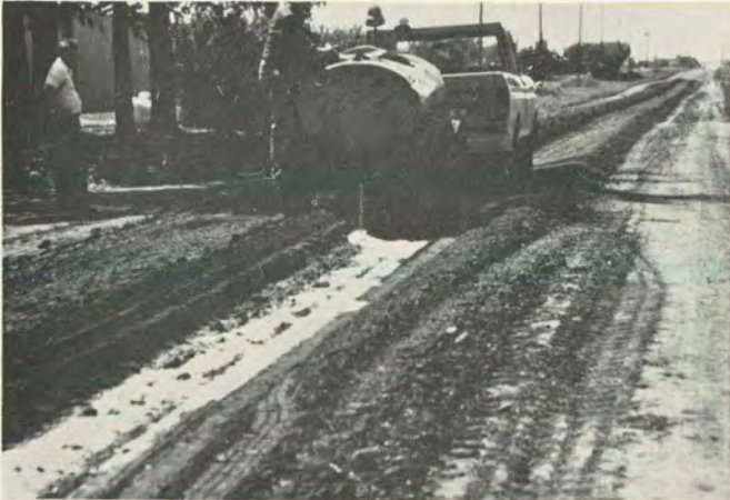
a. First stage application of Coherex to notched windrow.
