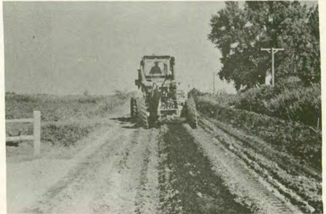
b. Initial blade grader mixing, section HC-2.
