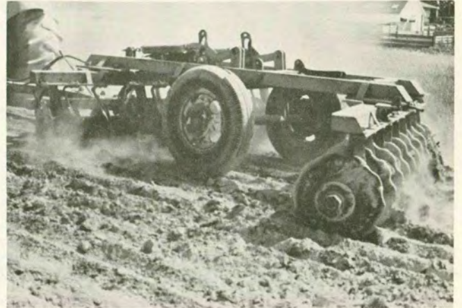
b. Initial mixing and pulverization of cement, fly ash and soil.
