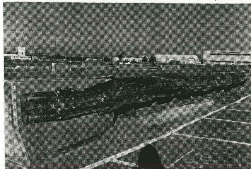
FIGURE 25. PHOTOGRAPHS OF DAMAGE TO APPROACH GUARDRAIL TRANSITION SECTION.
