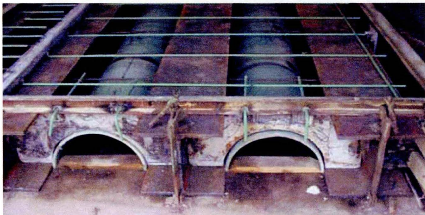
Transverse arches between the steel beams.
