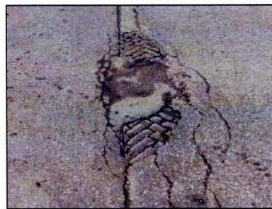
Asphalt Surface with Exposed Brick
