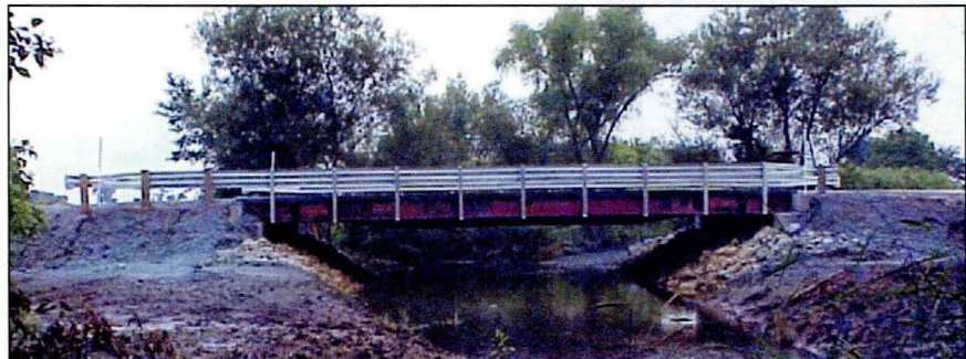
Finished Buchanan County RRFC Bridge
