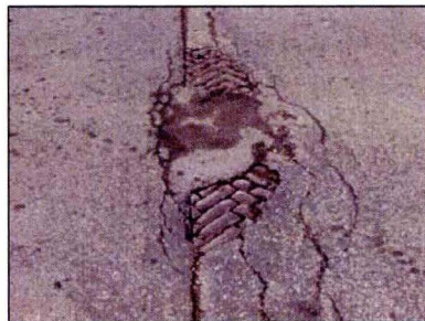
Asphalt Surface with Exposed Brick
