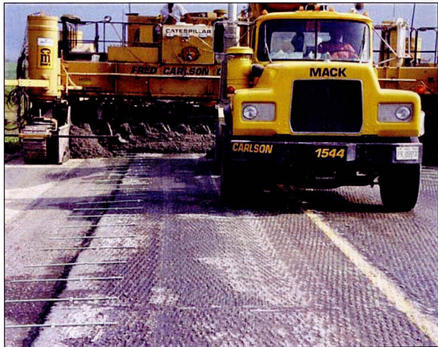
Stapled #4 bars that tie the widening unit to the thin overlay
