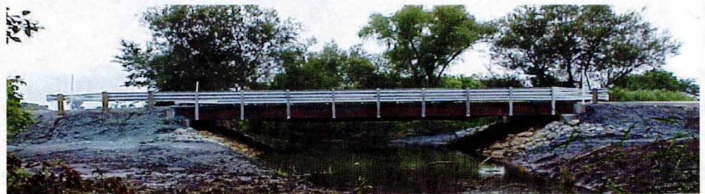
The finished Buchanan County RRFC Bridge
