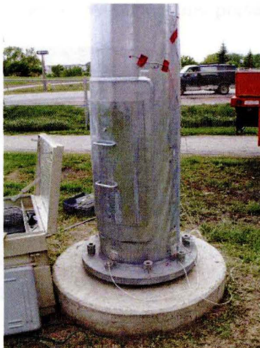
Replacement tower base
