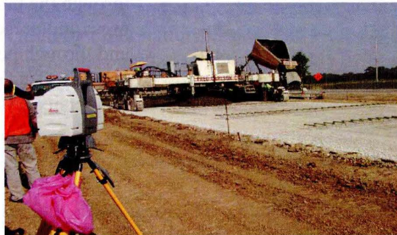
Performing laser scan on the subbase level
