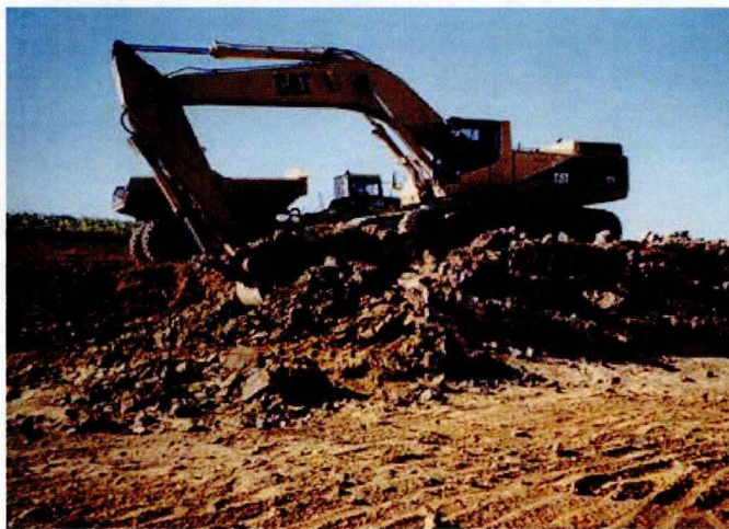
Soil mixing operation through layered soils, Des Moines, Iowa
