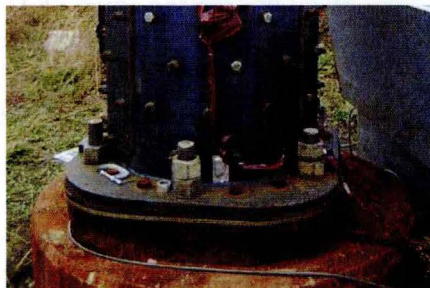
Bolted Reinforcing Jacket
