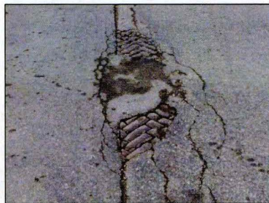
Asphalt Surface with Exposed Brick
