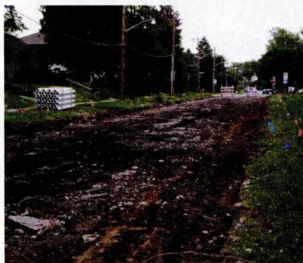
Existing non-uniform subgrade after pavement removal
