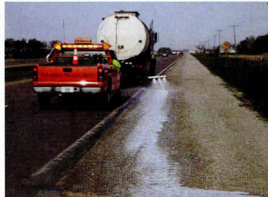
S.S. polymer typically applied to the granular shoulder
