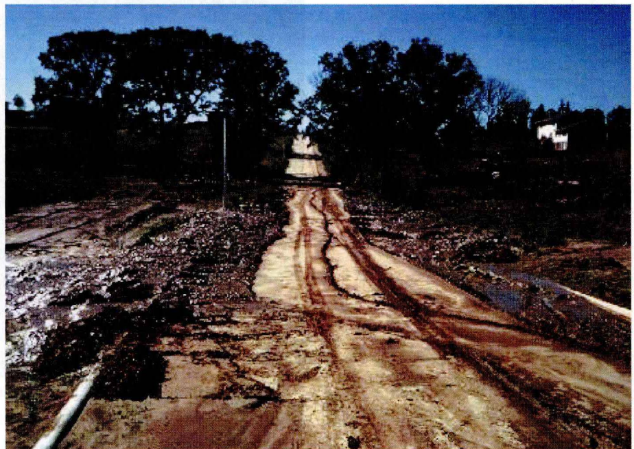
Sediment in street due to inadequate erosion and sediment control during construction - Photo: USDA NRCS Photo Gallery
