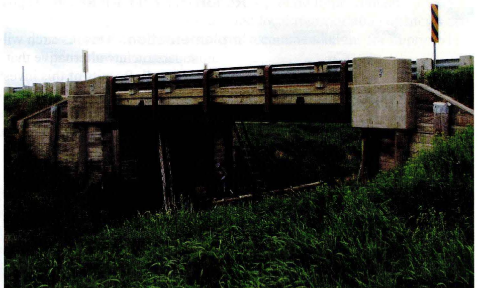
Evaluating the design of a steel bridge in Iowa
