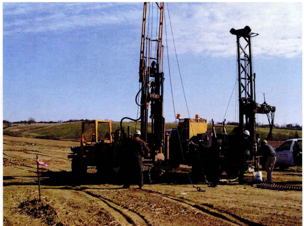
Cone Penetration Testing (setup on the left) and soil borings (right) in progress on the Crow Creek embankment. Photo: Thang Phan, Ph.D. candidate, Geotechnical Engineering, Iowa State University
