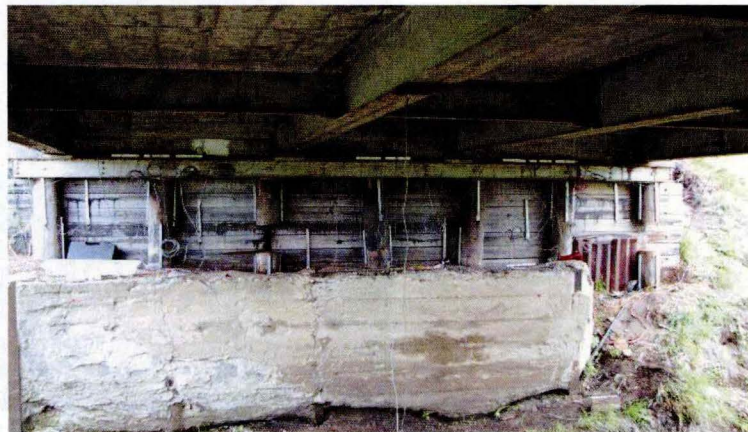
During removal of a bridge in Humboldt County, testing of the super- and sub-structure is made; instrumentation on the piling is visible.
