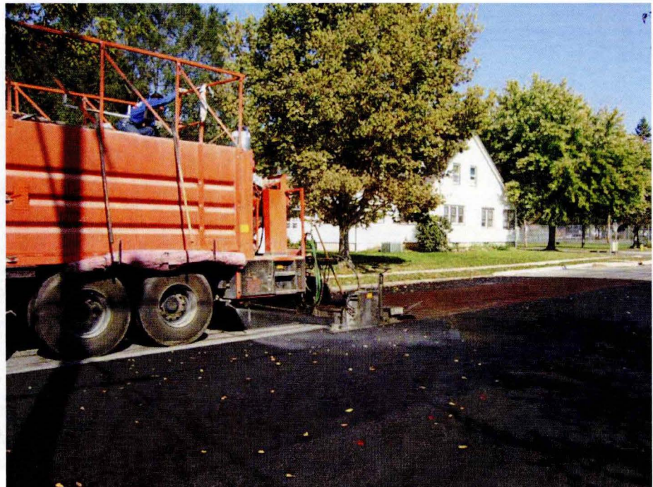
Micro-surfacing construction
