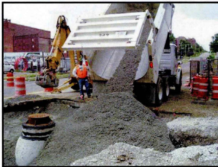
Large lift thickness used in utility cut trench backfilling Photo: Iowa State University/InTrans
