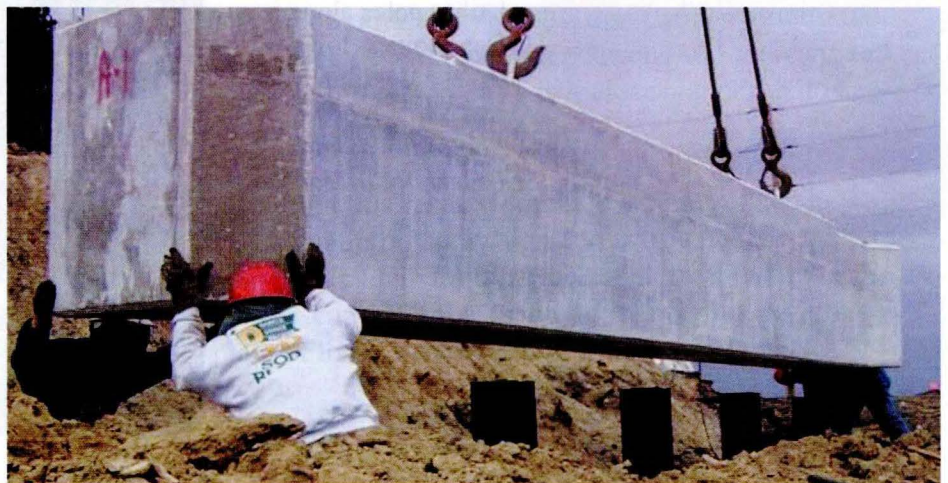
Boone County bridge substructure (West abutment) being placed Photos: Dr. Terry Wipf, Iowa State University/BEC
