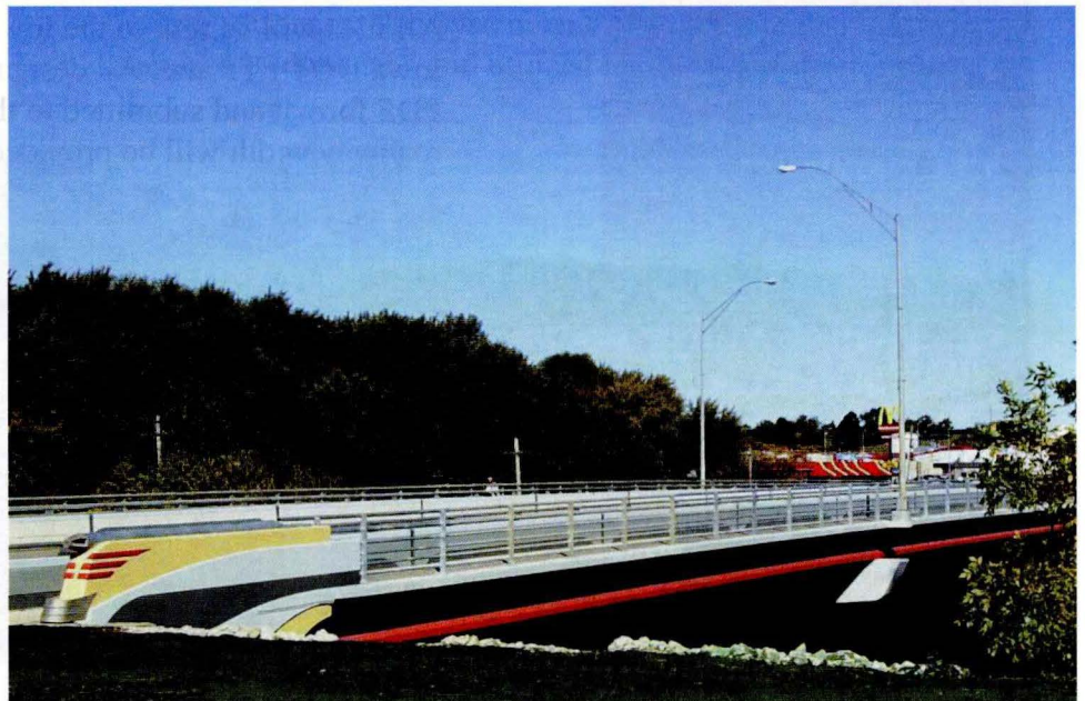
Three-span bridge on US 169 over the Des Moines River, Algona, IA Photo: WHKS & Company
