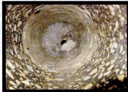
Rubblized PCC layer on IA-3 in Delaware County, Iowa
