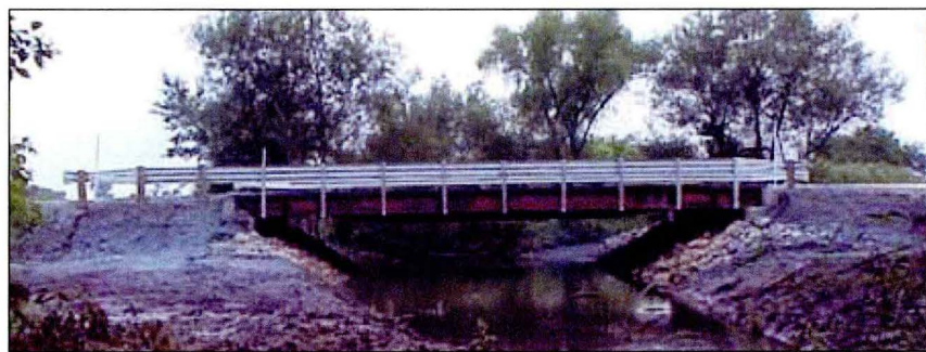
Finished Buchanan County RRFC Bridge
