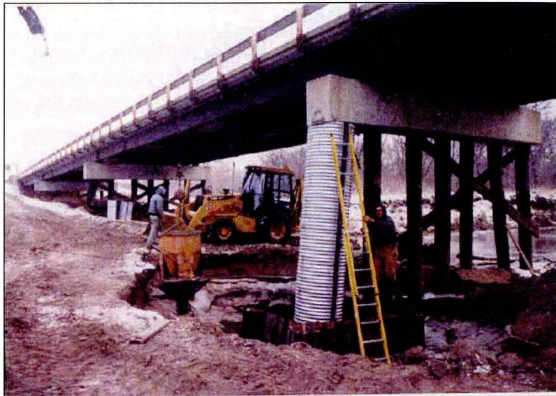
Jacking of Deteriorated Timber Piles
