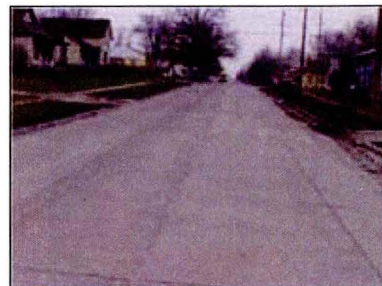
Completed Jointing Pattern
