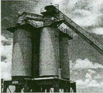
Stationary Five Bin Silo System
