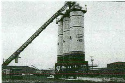
Slat Conveyor Feeding Silos
