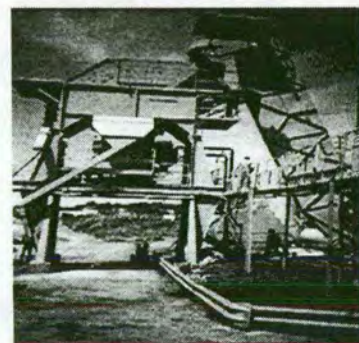
Angled Bucket Elevator Batch Plant
