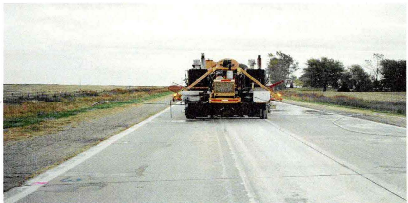
Surface grinder used in pavement rehabilitation
