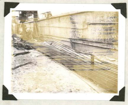
Drape strands or deflected strands are shown in the picture in a final position. These cables are normally partially stressed in a down position as shown in the diagram and raised to final position (shown by dashes) to complete the stressing operation.
