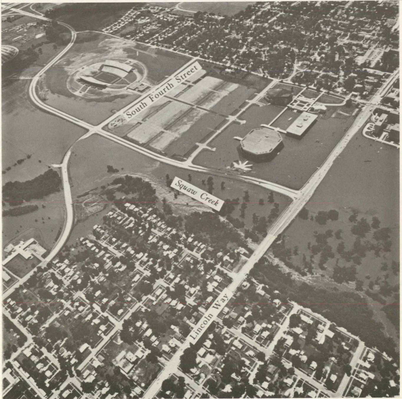
Figure 6. Squaw Creek flooding between South Fourth Street and Lincoln Way. 1427 hours.
