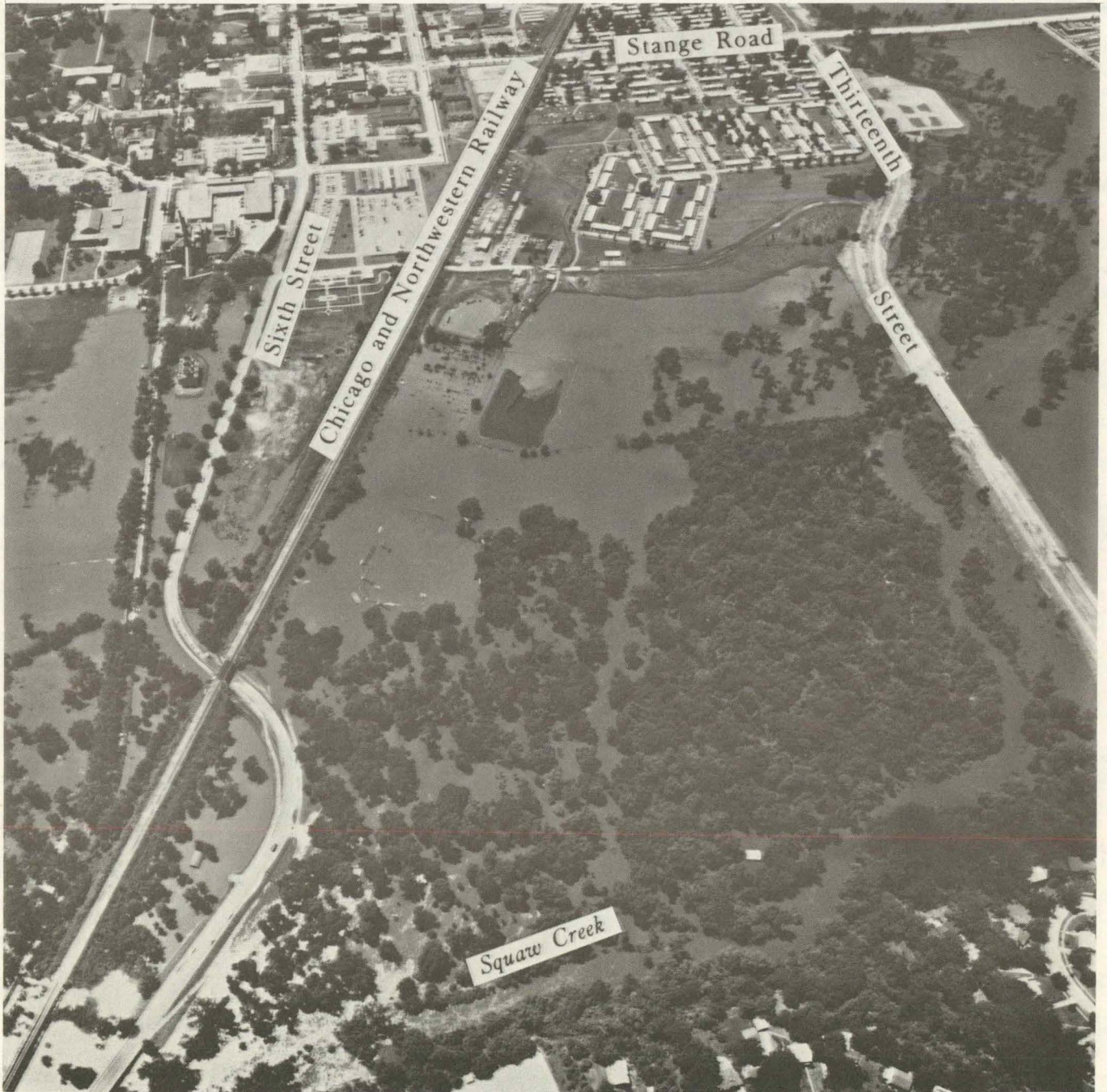
Figure 8. Squaw Creek flooding between Sixth Street and Thirteenth Street. 1426 hours.
