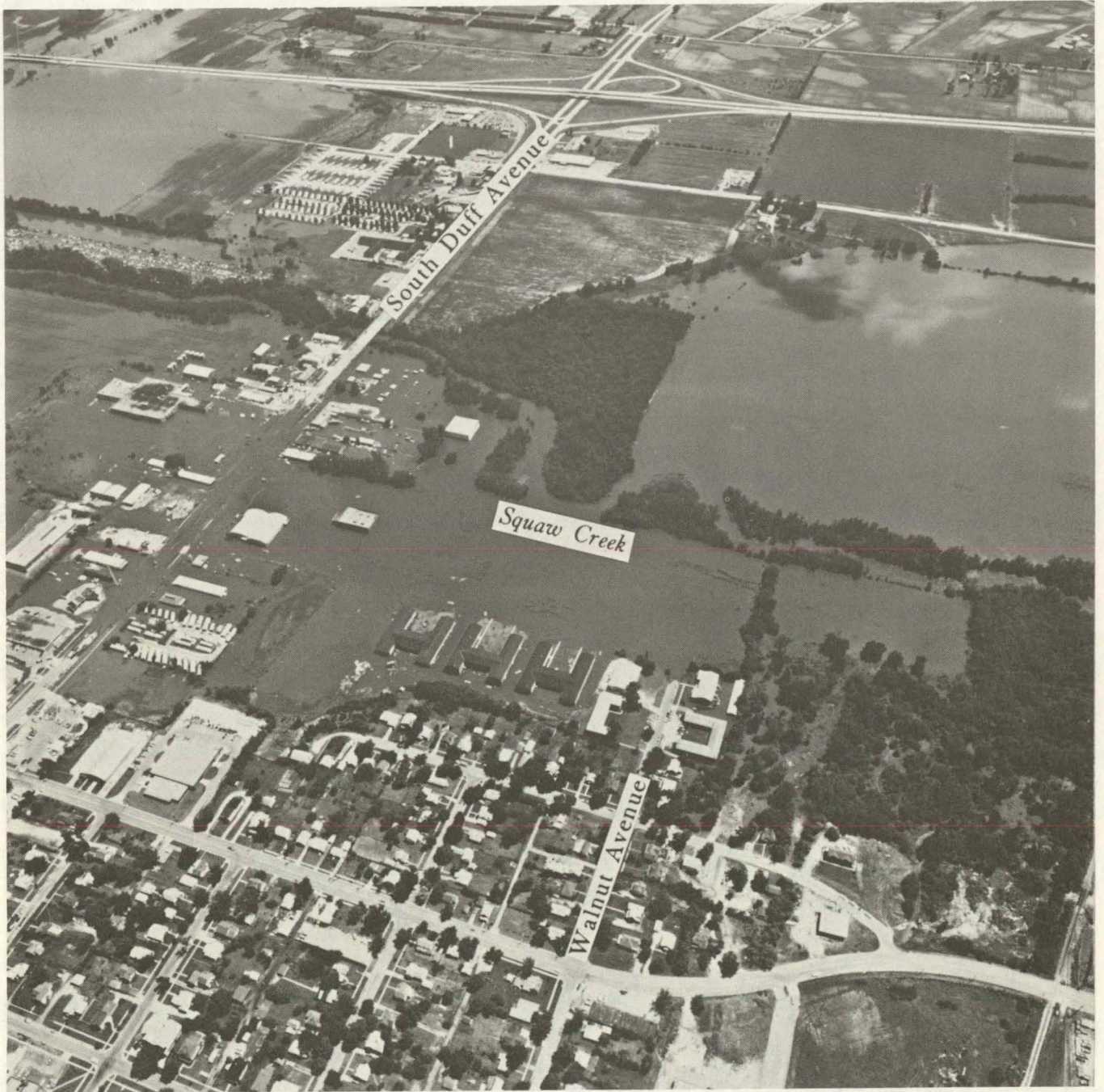
Figure 4. Squaw Creek flooding between South Duff and Walnut Avenues. 1428 hours.
