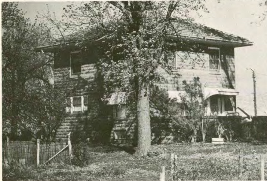
STRUCTURE CL17: EARLY EXAMPLE OF TWO STORY CONCRETE BLOCK HOME CONSTRUCTION
