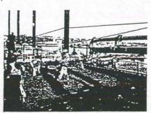
Concrete placement for the last slab in the truss unit was completed in September
