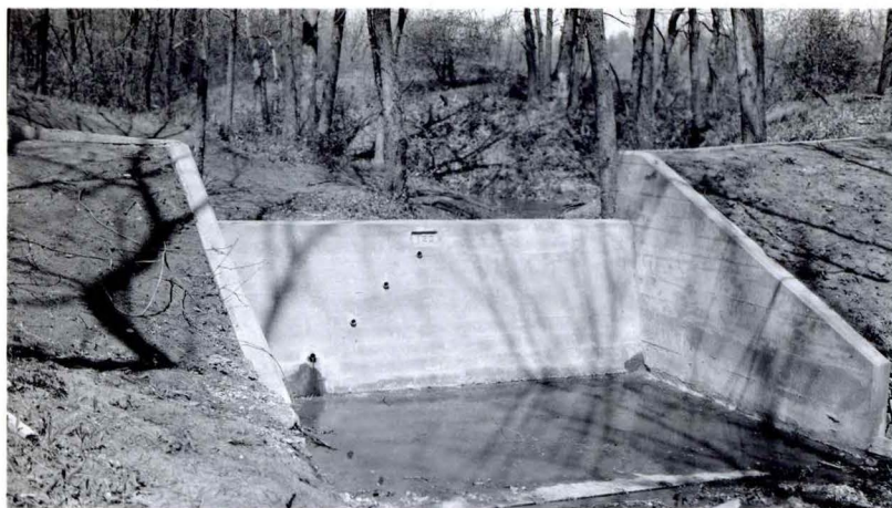
Lake Wapello Screen & Log Boom at Spillway
