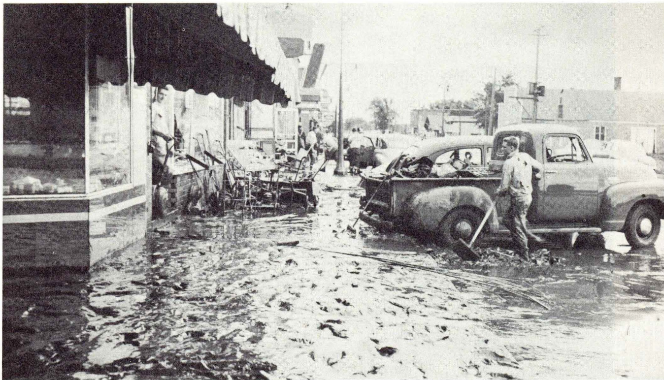
Figure 5. --Thick mud deposits left by the Floyd River in suburban Leeds. Photograph by George Newman, Sioux City, Iowa.
