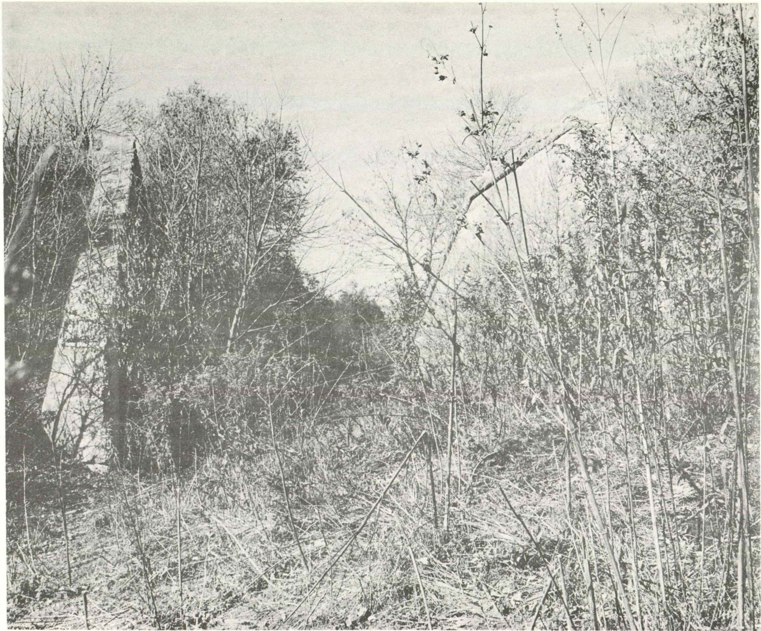
Photo No. 10. Former underpass for second abandoned railroad, and proposed location for culvert spillway for Railroad Lake.
