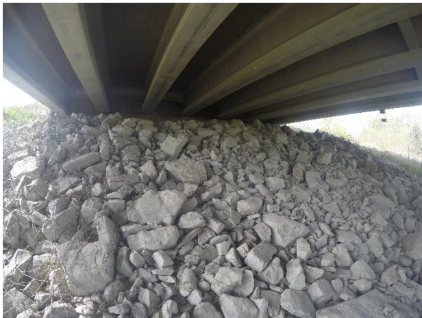
Figure 31. Undersized loose riprap in Madison County, Iowa
