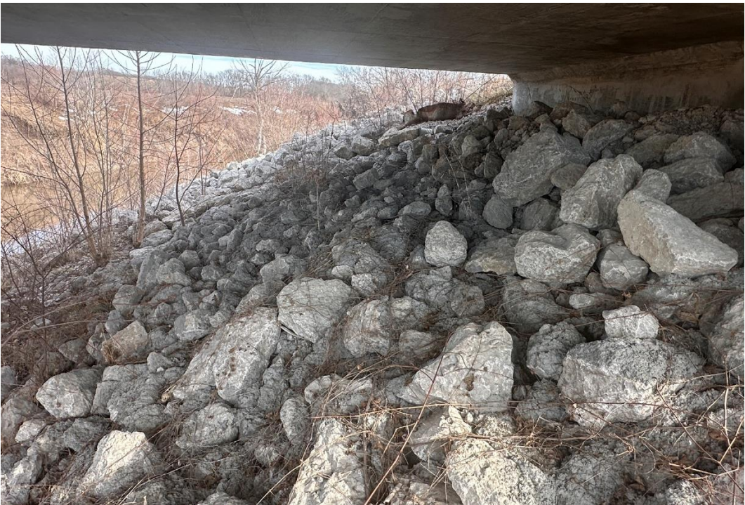
Figure 47. Wayne County Pilot installation as of February 2024
