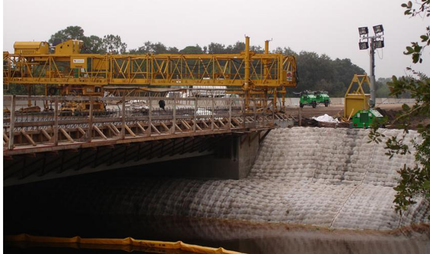
Figure 12. Grout-filled mattresses after installation
