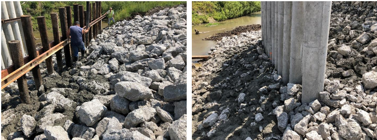
Figure 41. Wayne County pilot installation grouting
