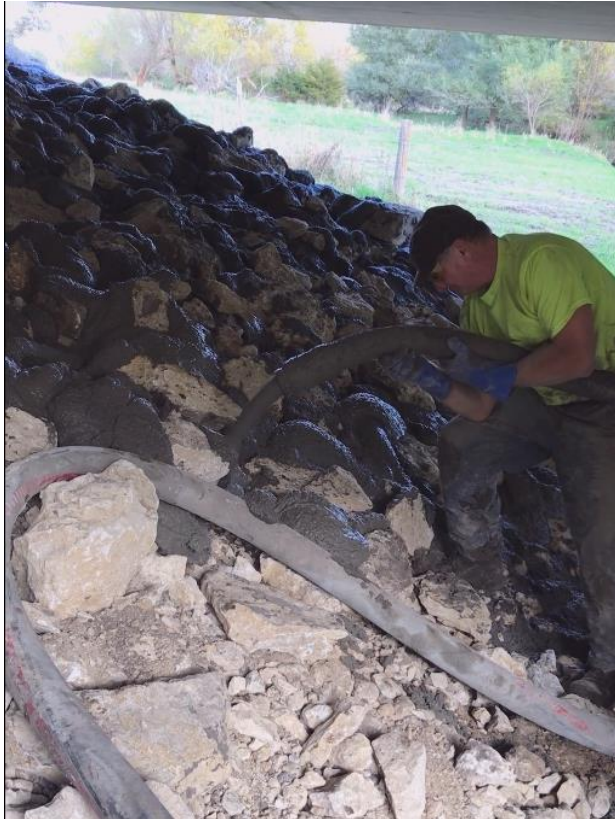
Figure 35. Grout placement of FHWA mix (left) and Buchanan County grout (right)
