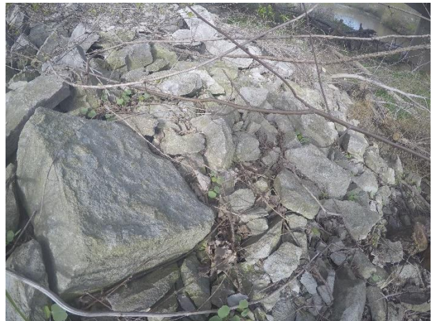
Figure 31. Undersized loose riprap in Madison County, Iowa
