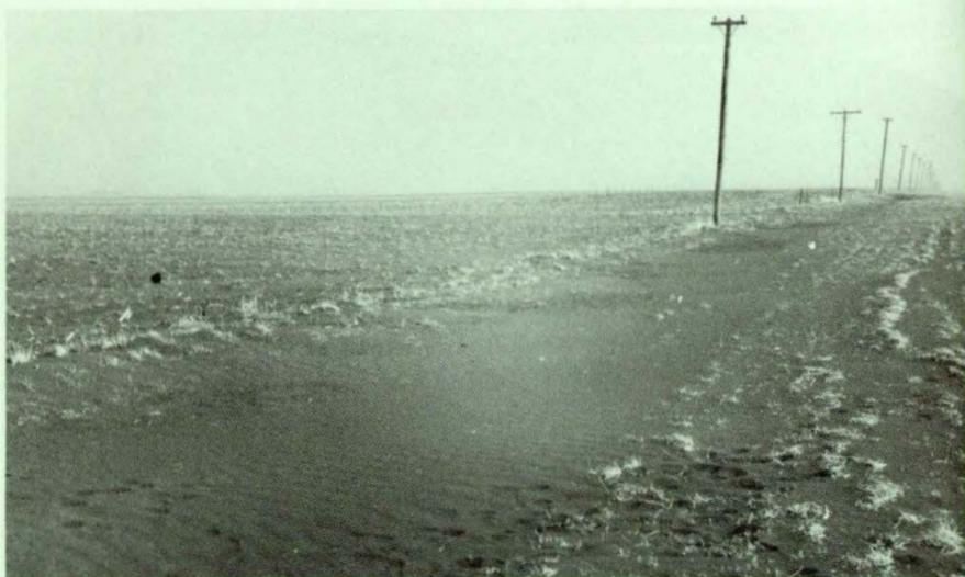
*Problem — Wind erosion with road ditch filled with soil from a nearby bean field which had been fall plowed.*
