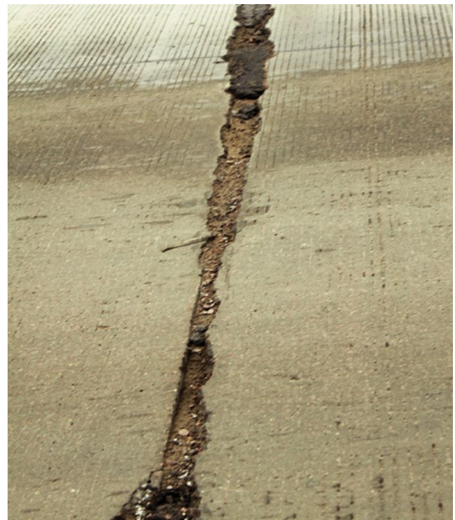
Figure 6-34. Joint damage
