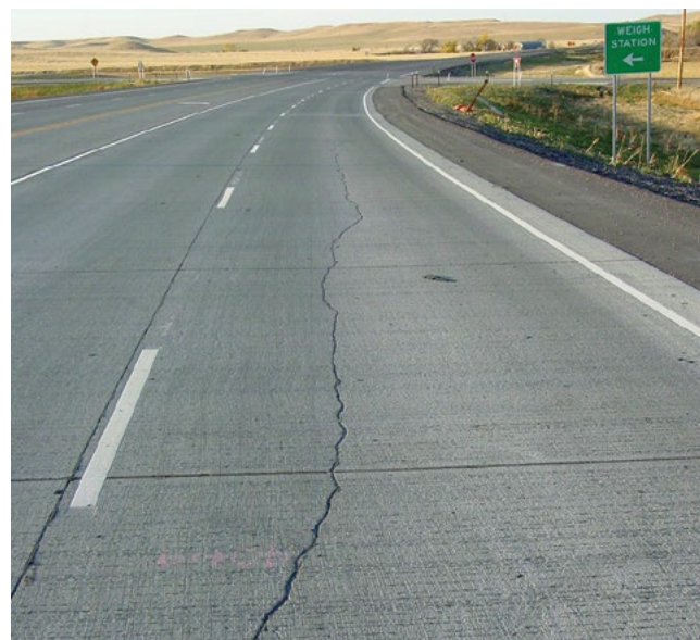
Figure 3-7. Structural longitudinal crack
