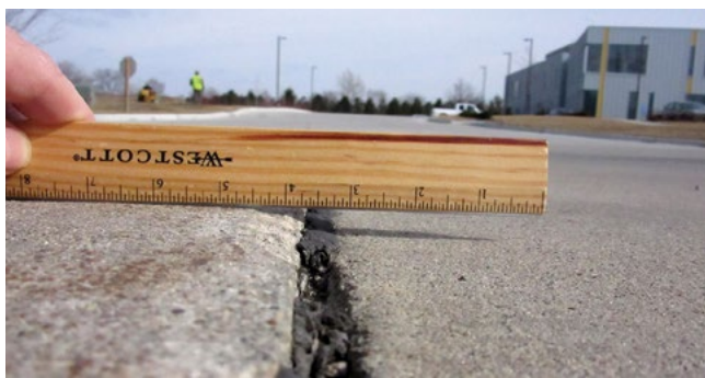
Figure 3-9. Faulting
