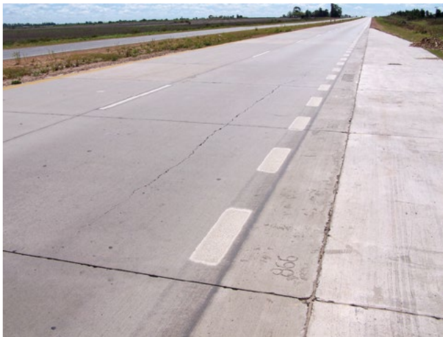
Figure 6-29. Random longitudinal crack
