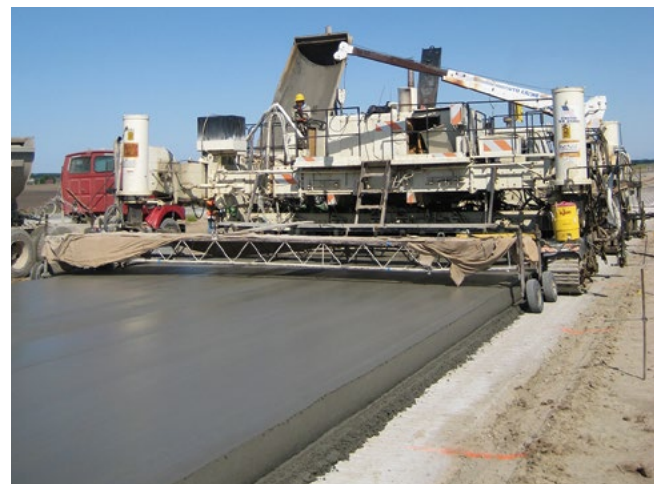
Figure 8-5. Trackline of slipform paving machine
