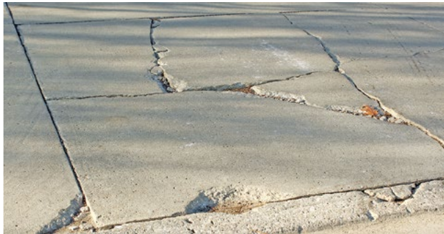
Figure 3-8. Shattered slab
