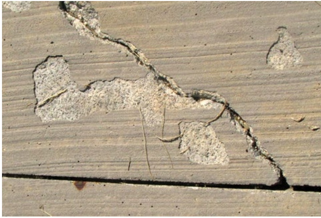
Figure 6-35. Scaling
