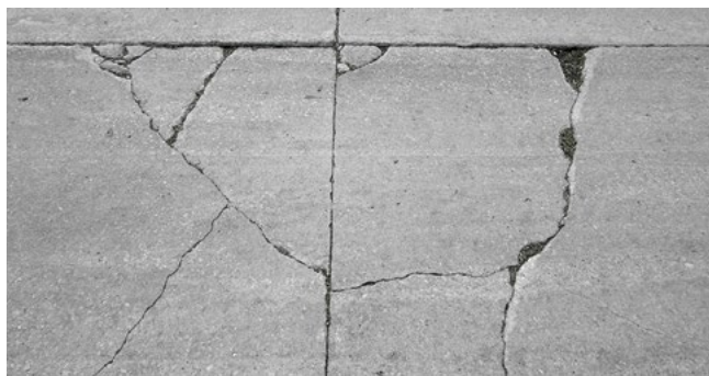
Figure 6-30. Corner break
