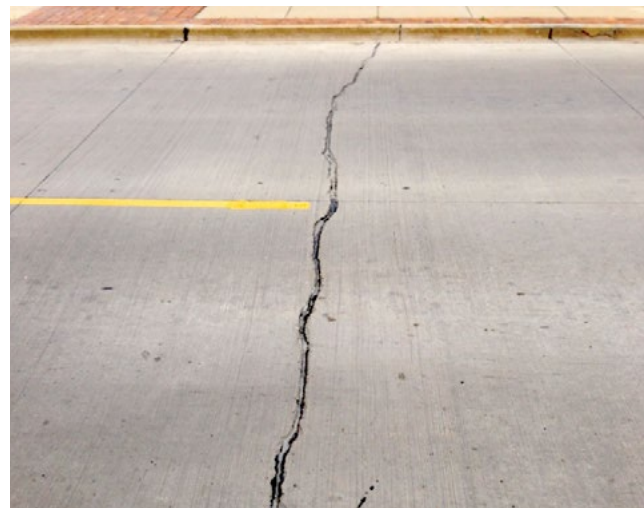
Figure 3-6. Structural transverse crack
