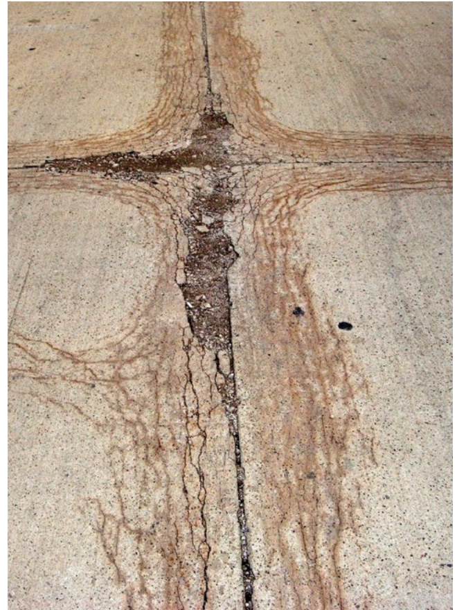
Figure 6-36. D-cracking
