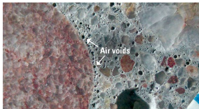
Figure 5-29. A typical example of air voids clustered around an aggregate particle
