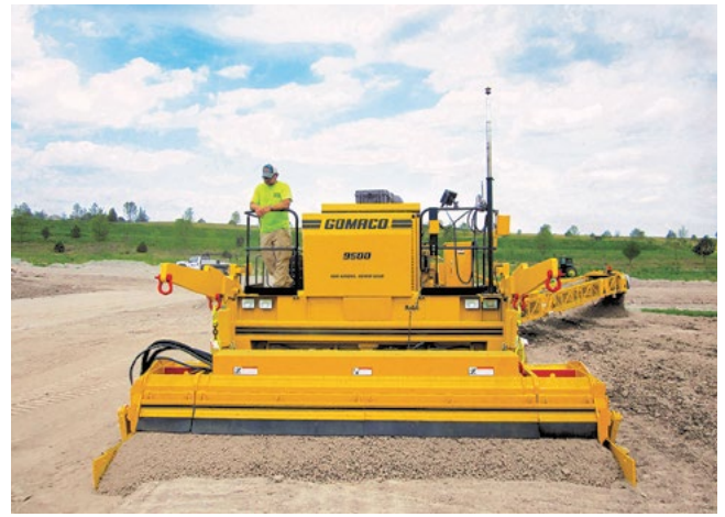
Figure 8-3. Trimming subgrade material
