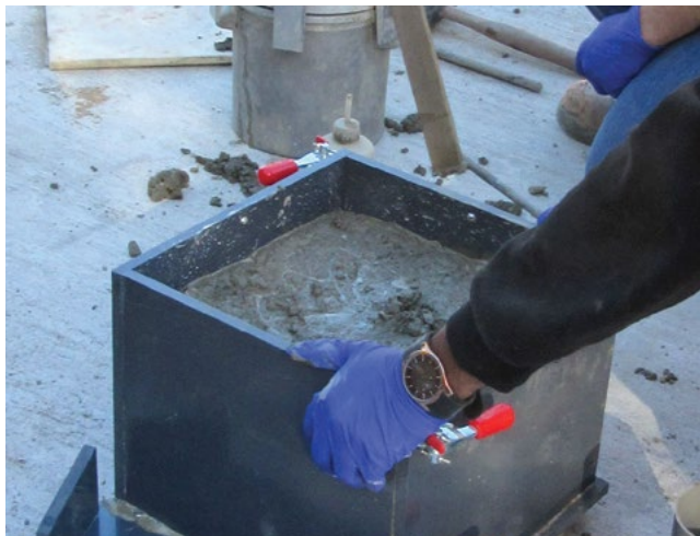
Step 3 Insert vibrator downward for 3 seconds and upward for 3 seconds. Remove vibrator.
