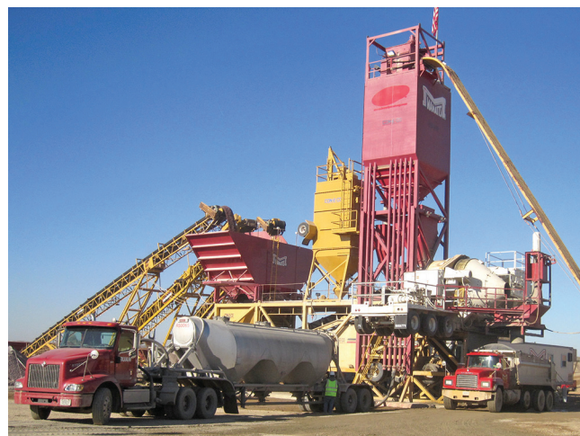
Jim Grove, ATI Inc./FHWA, used with permission
