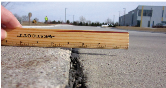
Figure 3-9. Faulting
