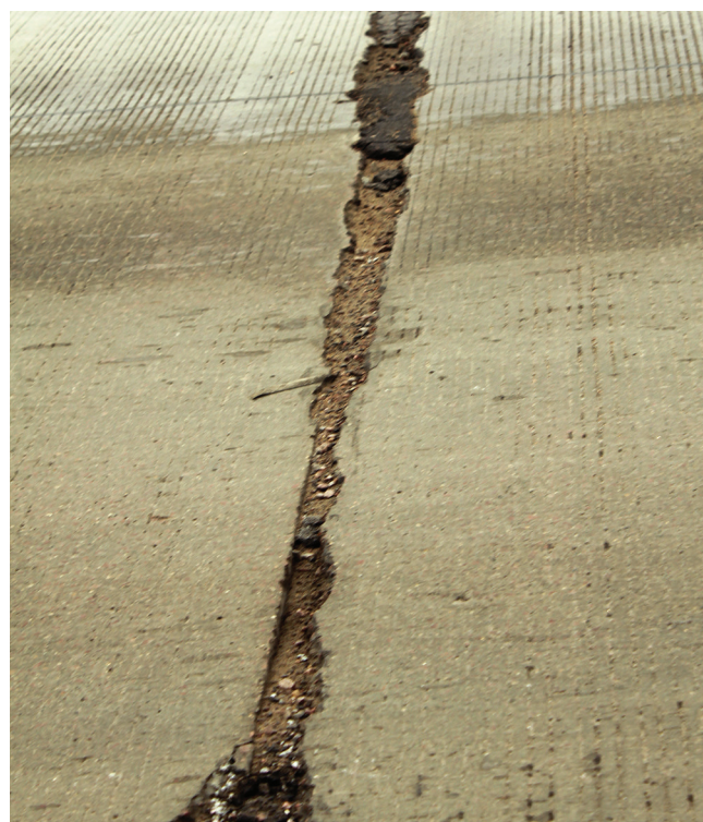
Figure 6-34. Joint damage
