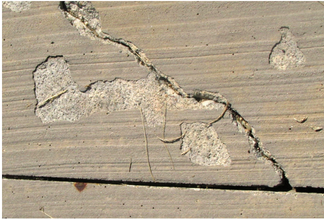
Figure 6-35. Scaling
