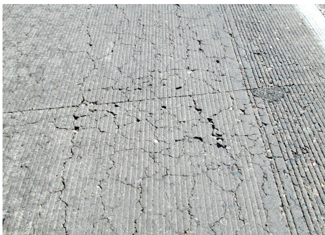
Figure 6-27. Map cracking
