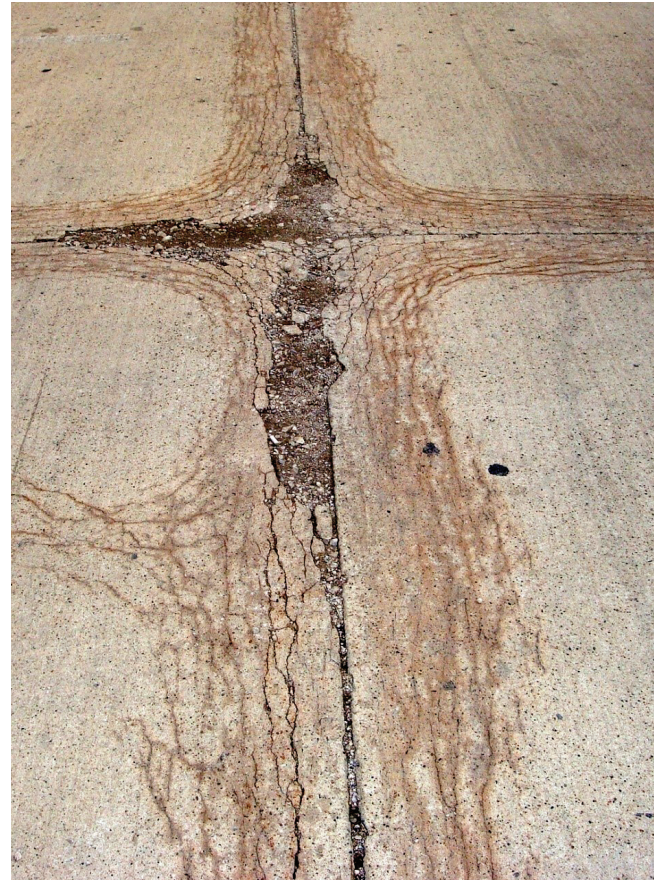
Figure 6-36. D-cracking
