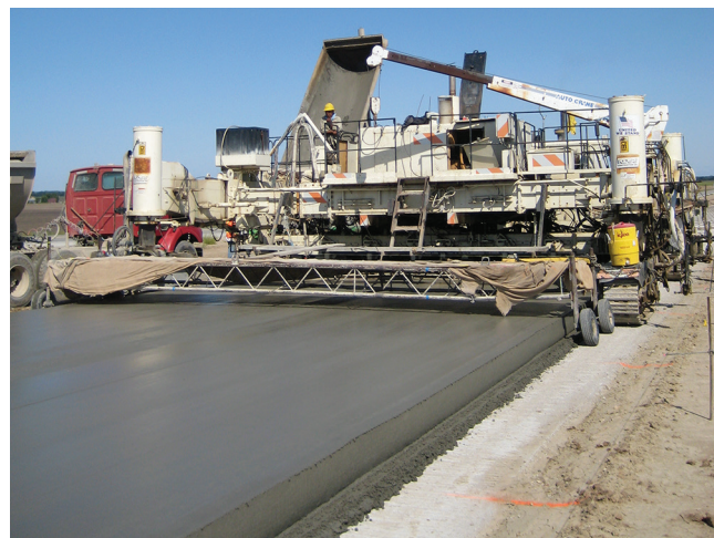
Figure 8-5. Trackline of slipform paving machine
