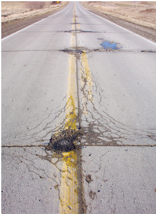
Jim Grove, ATI Inc./FHWA, used with permission
