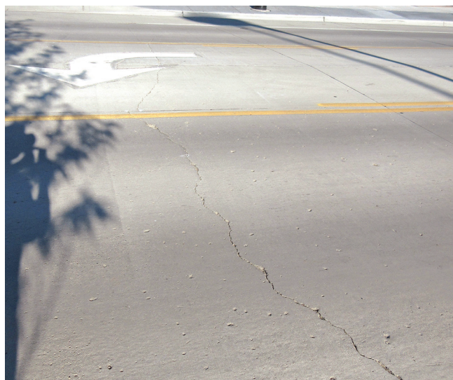
Jim Grove, ATI Inc./FHWA, used with permission
