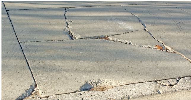
Figure 3-8. Shattered slab
