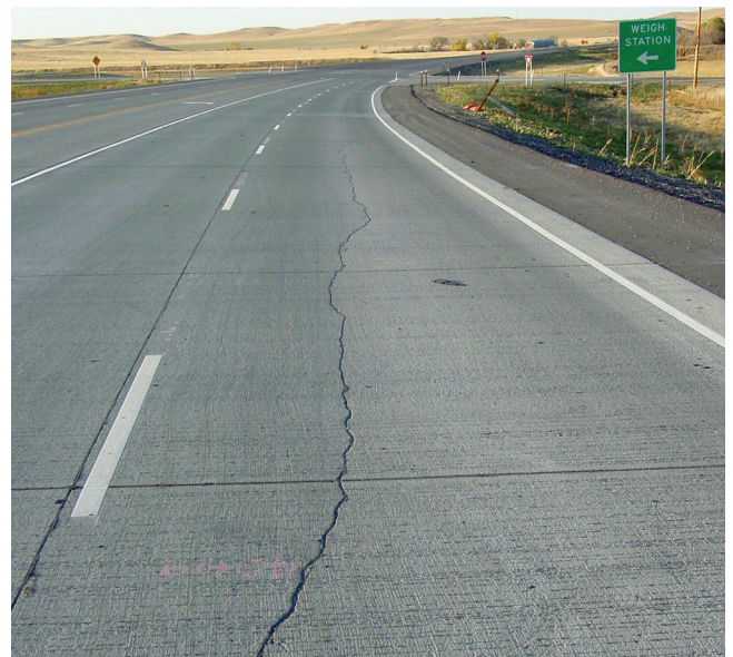
Figure 3-7. Structural longitudinal crack
