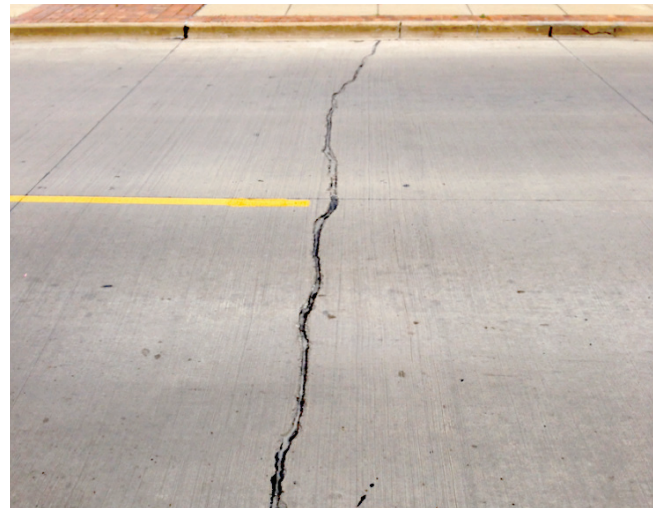
Figure 3-6. Structural transverse crack
