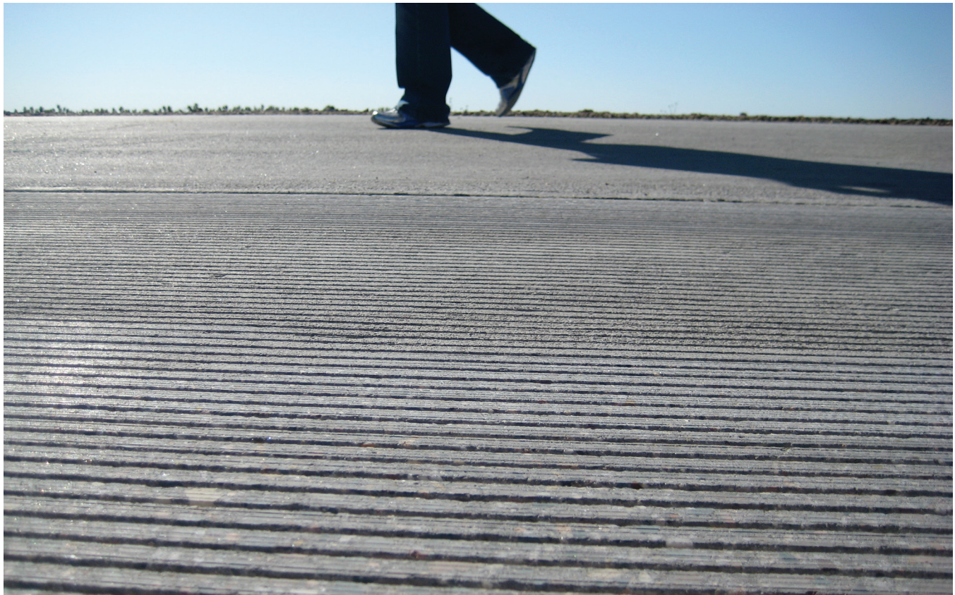
Figure 3-11. Next-generation concrete surface (NGCS)
