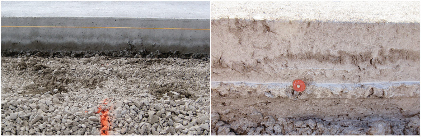
Figure 8-20. Dowel basket marked with paint for the saw crew (left) and an inserted dowel marked with a nail and washer (right)
