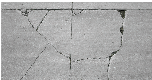
Figure 6-30. Corner break
