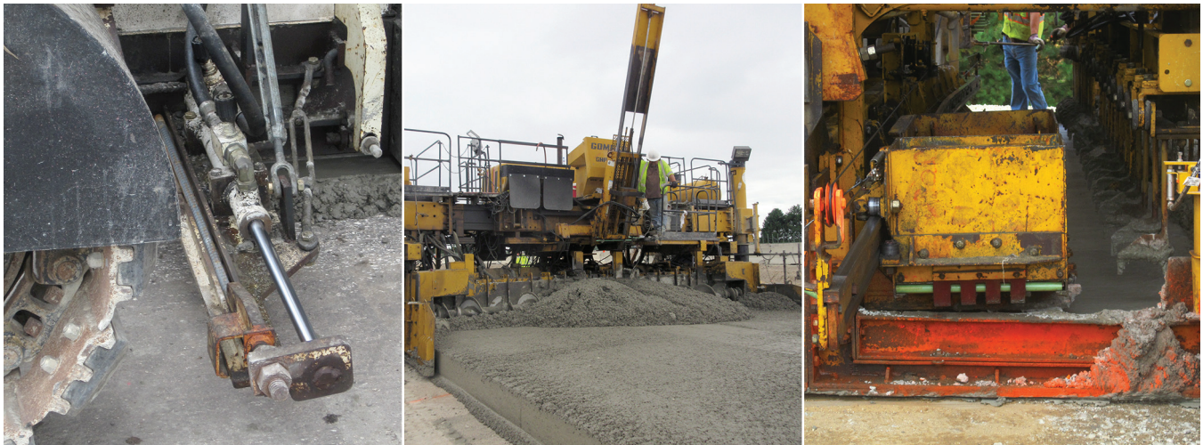
Jim Grove, ATI Inc./FHWA, used with permission
