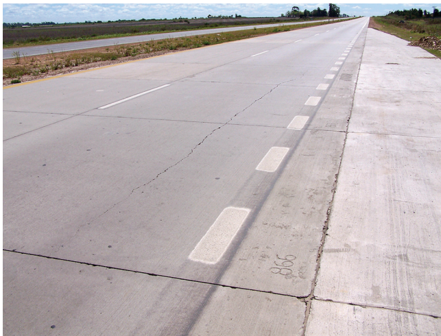
Figure 6-29. Random longitudinal crack
