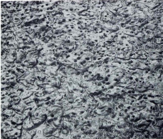
Fig. 5. Exposed portion of a guard gate raised from the bottom of the Mississippi River showing the nymphal burrows of Hexagenia bilineata .
