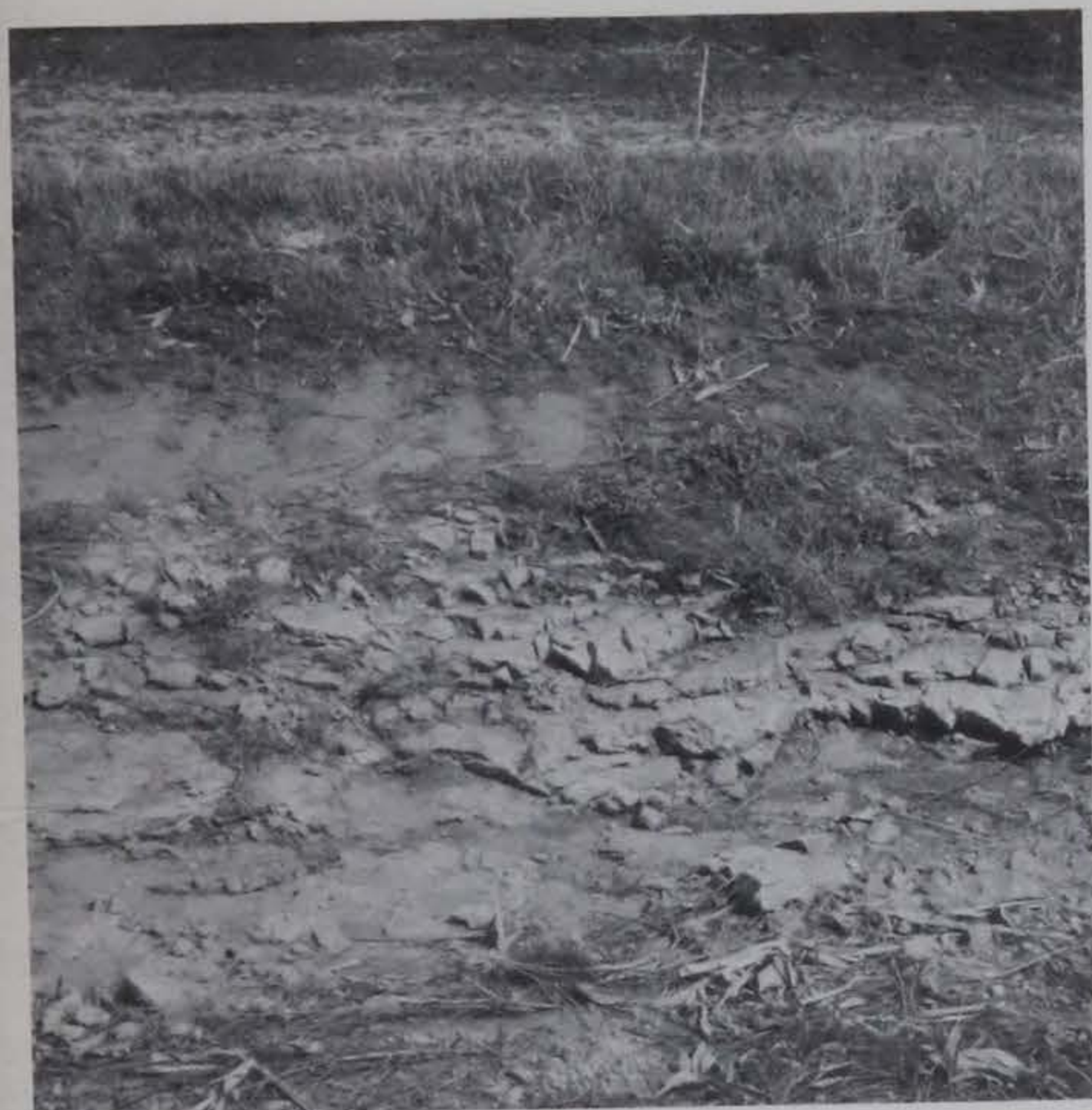
Figure 15.—Fractured limestone is too near the surface for filtering and purification of effluent.
