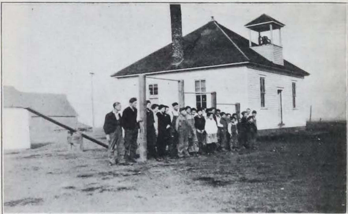
Center District No. 4, Bloomington Township, Decatur County.
